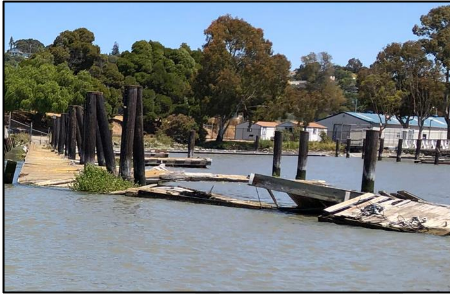
Figure 4: Existing Condition of A-Dock
