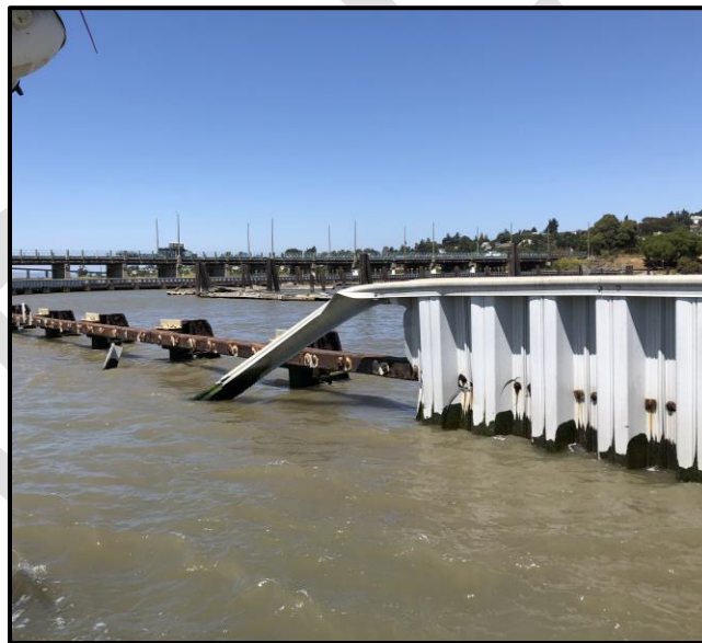
Figure 6: Existing Conditions at Sheet Pile Wall
