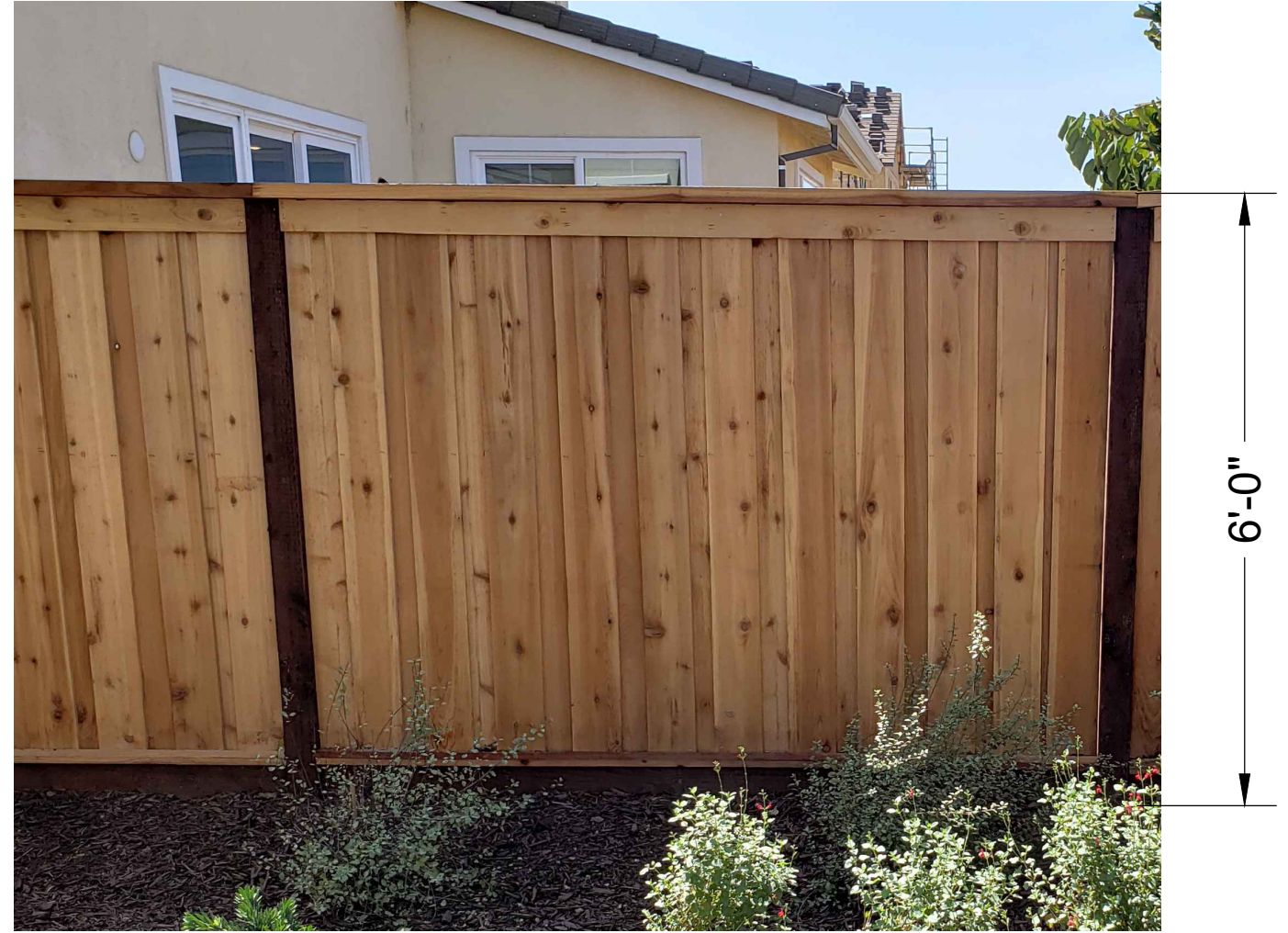
A GOOD NEIGHBOR FENCE 6' HIGH WOOD FENCE AT PRODUCTION HOMES
