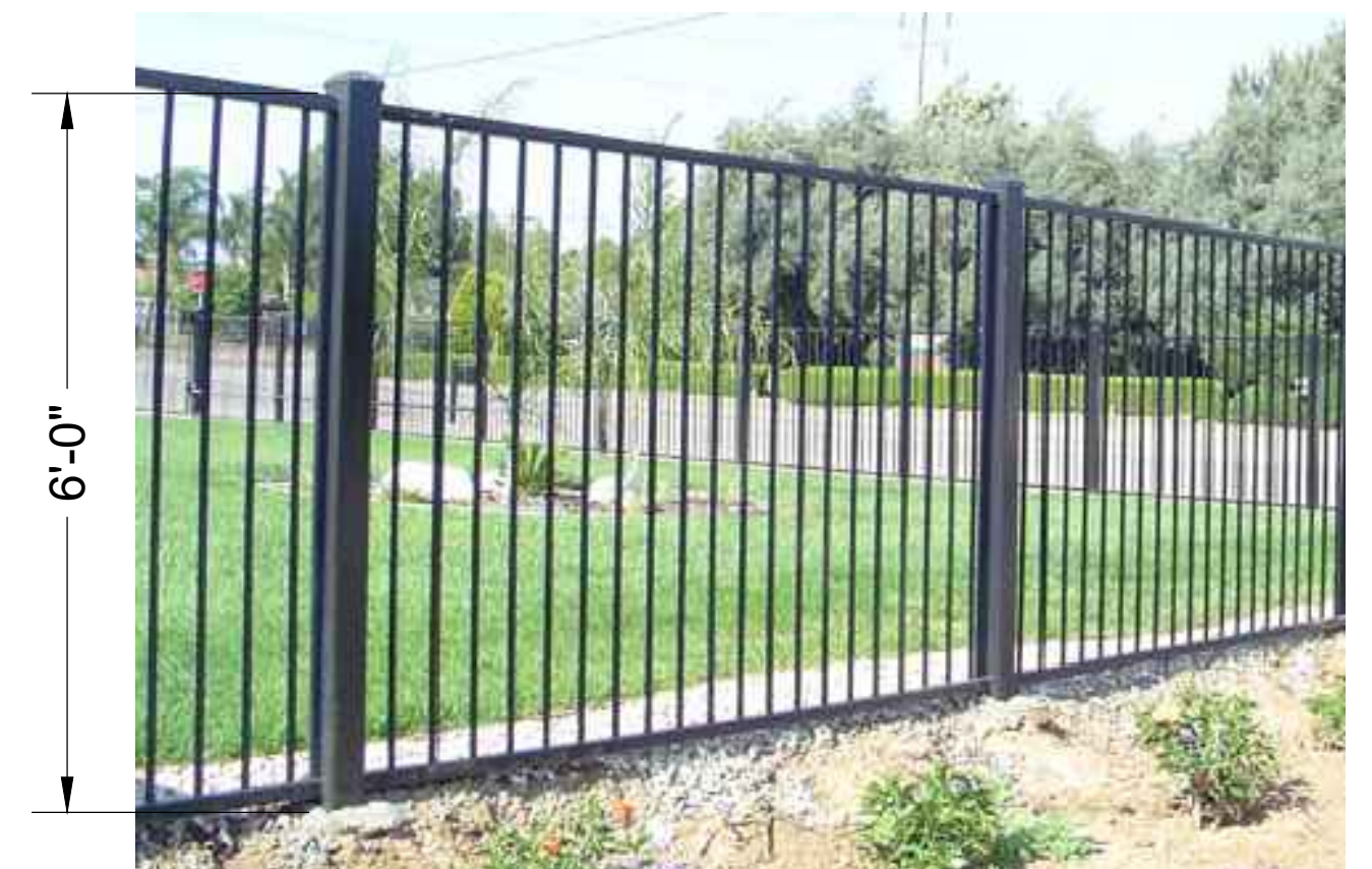
B VIEW FENCE 6' HIGH TUBE STEEL AT PRODUCTION HOMES
