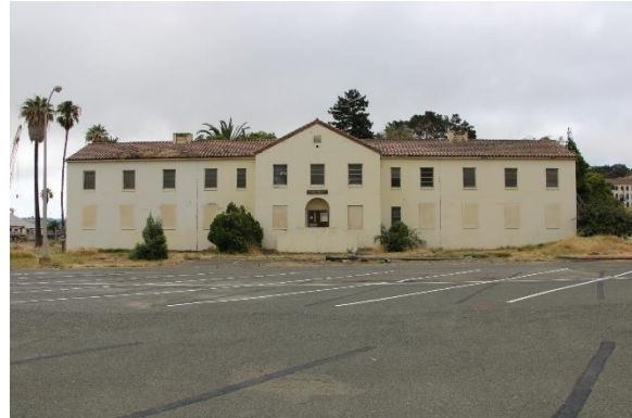
Photograph 6 Building H79 North Elevation, View South
