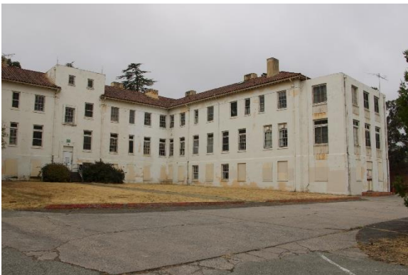
Photograph 3 Building H73 East and South Elevations, View Northwest
