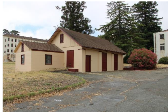
Photograph 4 Building H34 North and East Elevations, View Southwest
