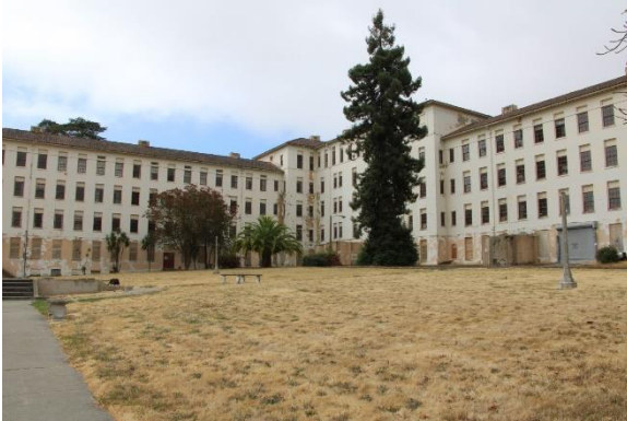
Photograph 1 Building H72 East and South Elevations, View Southwest
