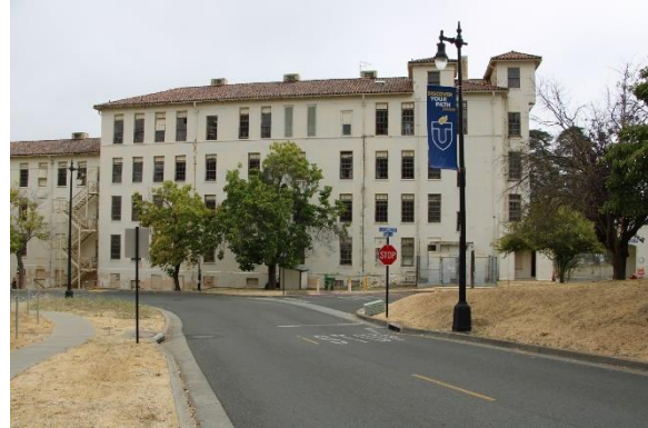
Photograph 2 Building H72 West Elevation, View East
