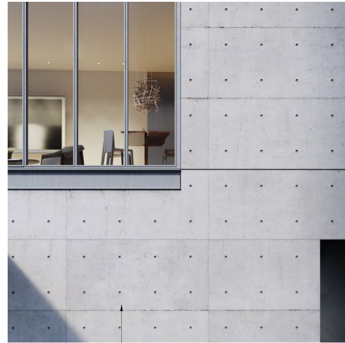
POURED IN PLACE CONCRETE
