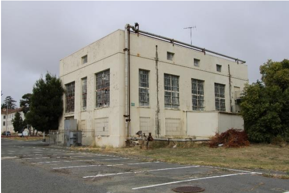
Photograph 5 Building H74 West and South Elevations, View Northeast
