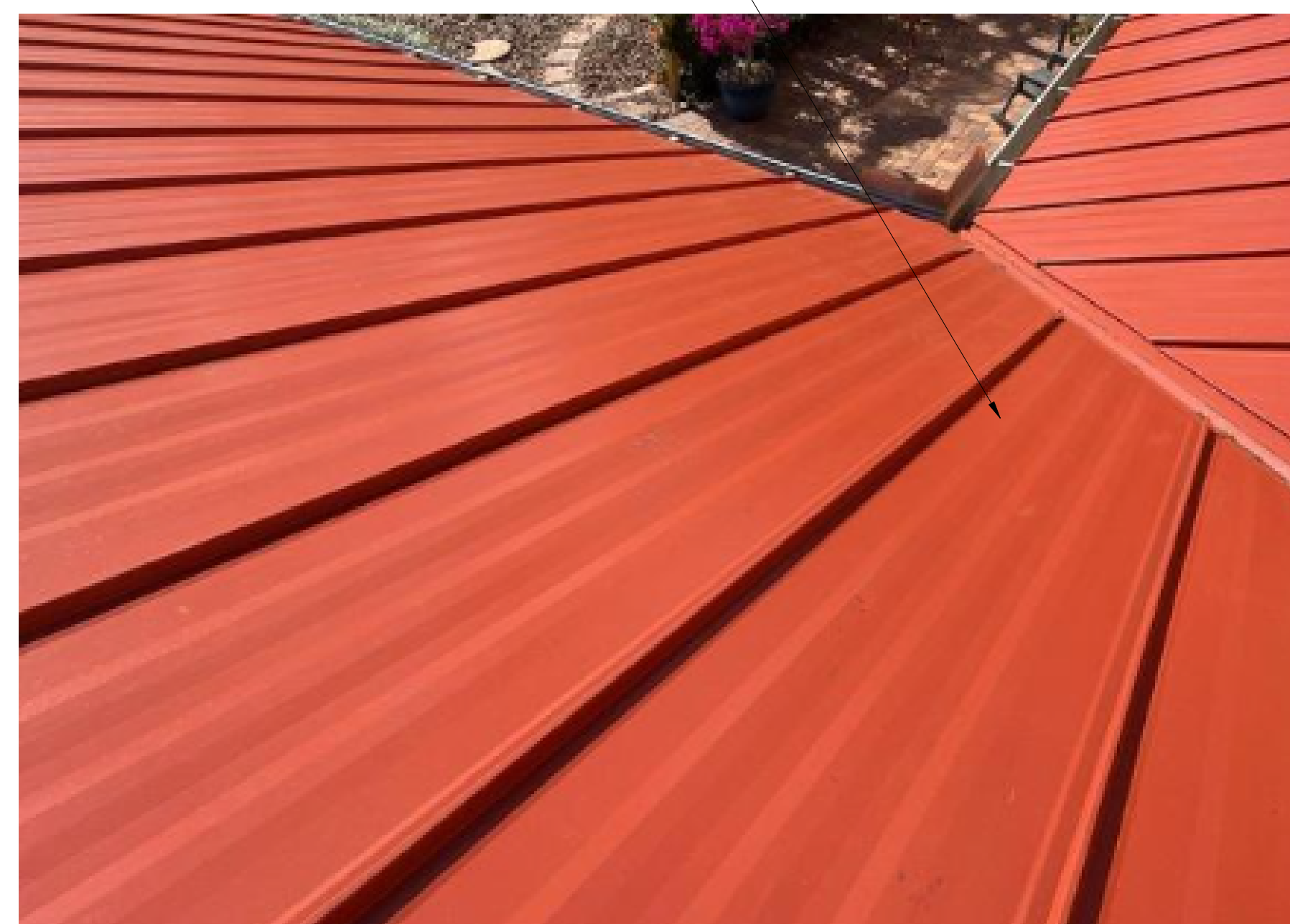
TMP- VERSA-SPAN™ STRUCTURAL SNAP-LOCK PROFILE: STRIATIONS 24 GAUGE KYNAR 500® PAINTED STEEL G-90 GALVANIZED OR AZ-50 TERRA COTTA SRI-43
