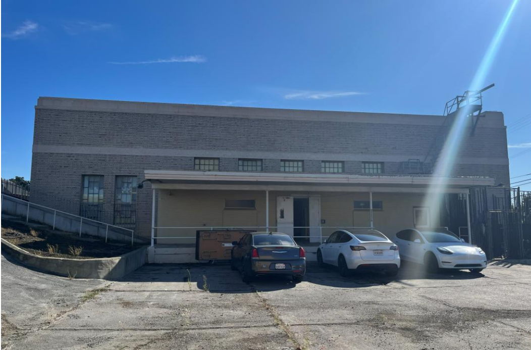
Photograph 4: Subject property showing west façade with loading dock, camera facing east .
