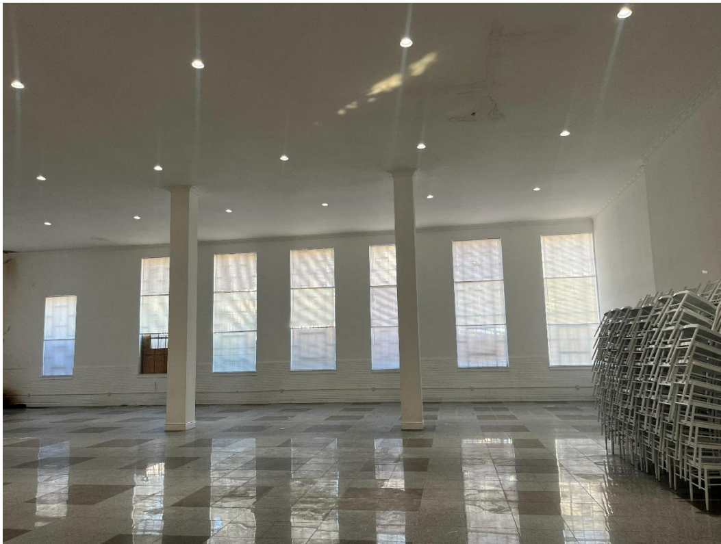
Photograph 9: Subject property lobby showing former workroom, camera facing north .
