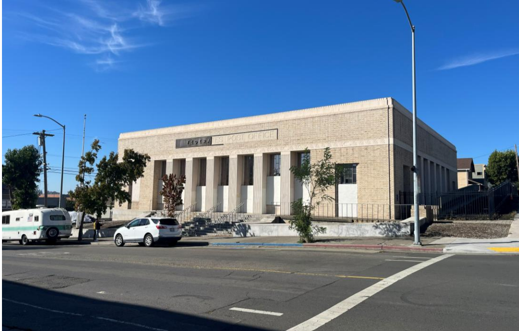
Photograph 2: Vallejo Post Office from across the street showing primary (east) and north facades, camera facing west.
