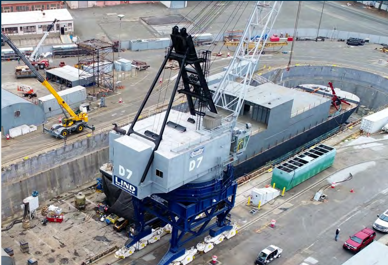
Lind Marine Completes Waterborne Data Center Barge Project on the Mare Island Naval Complex in Vallejo, CA
