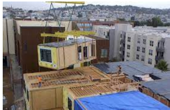
Source: Factory OS, City of Vallejo
