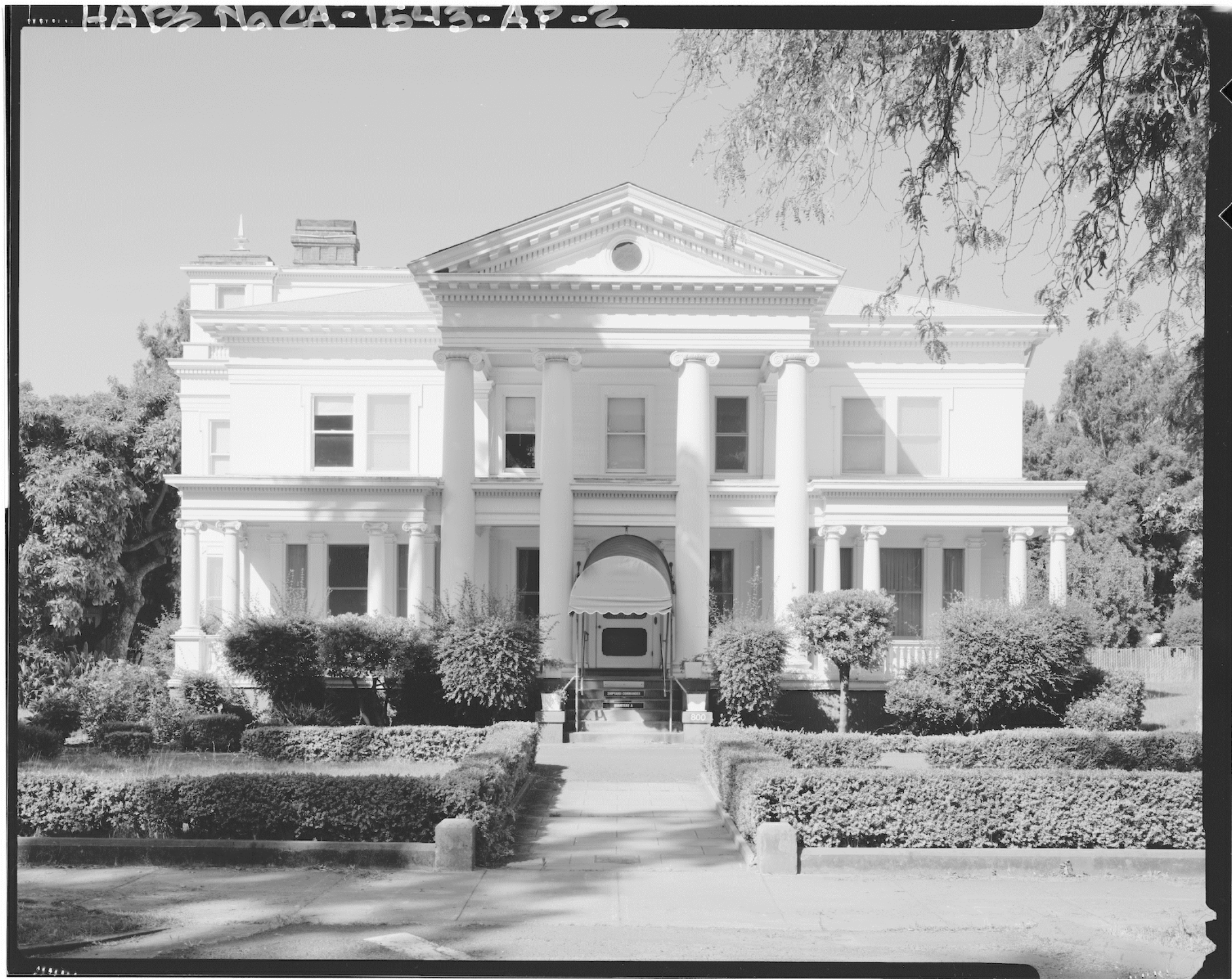
18 EAST ELEVATION - HABS
