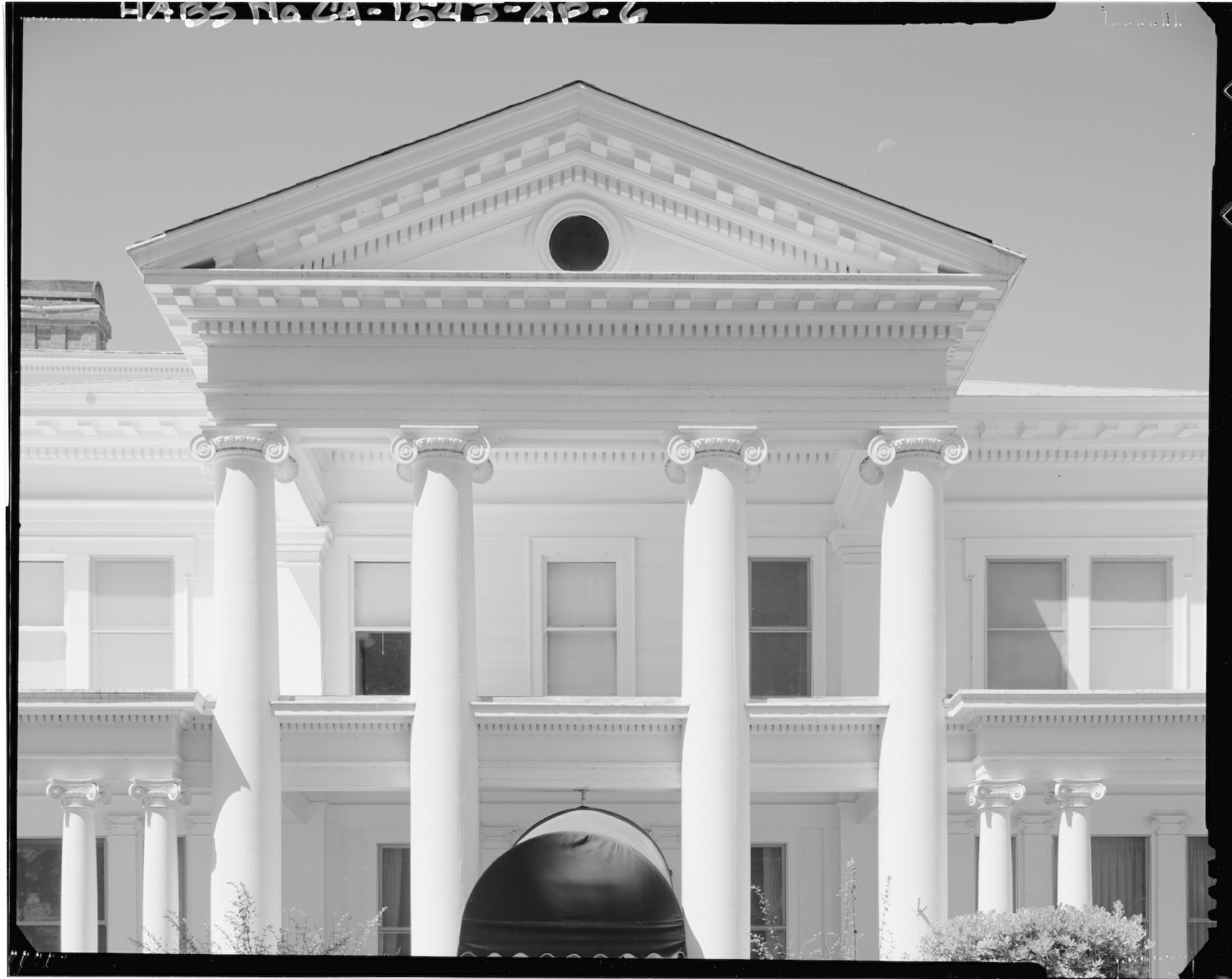
10 EAST ELEVATION - HABS
