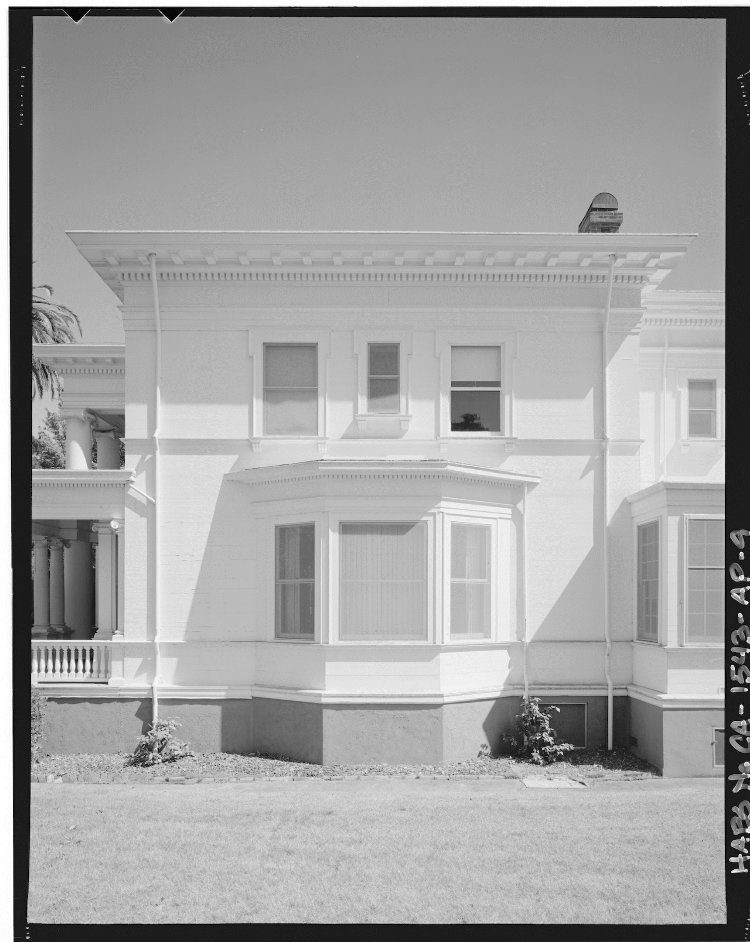
12 NORTH ELEVATION - HABS
