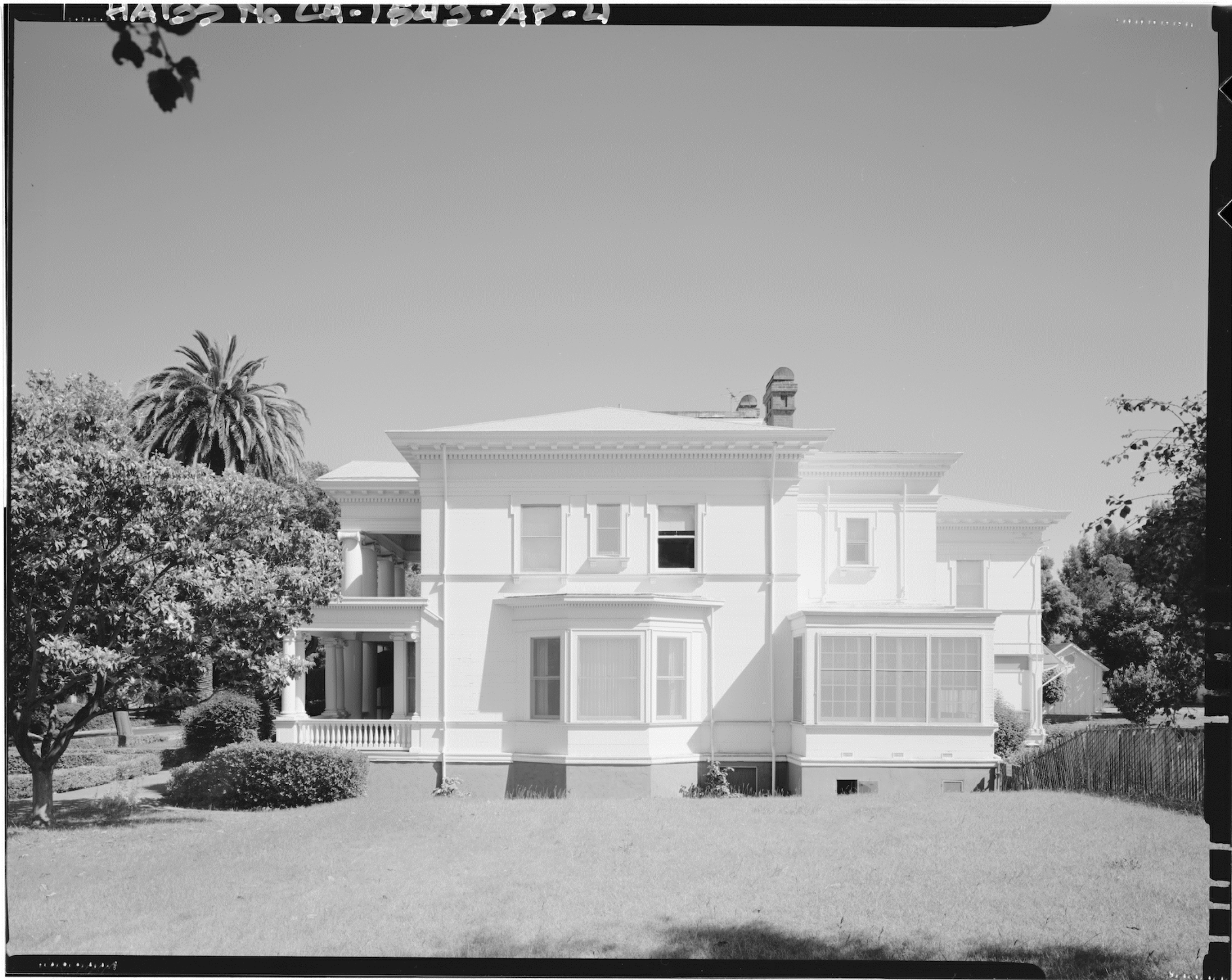
20 NORTH ELEVATION - HABS
