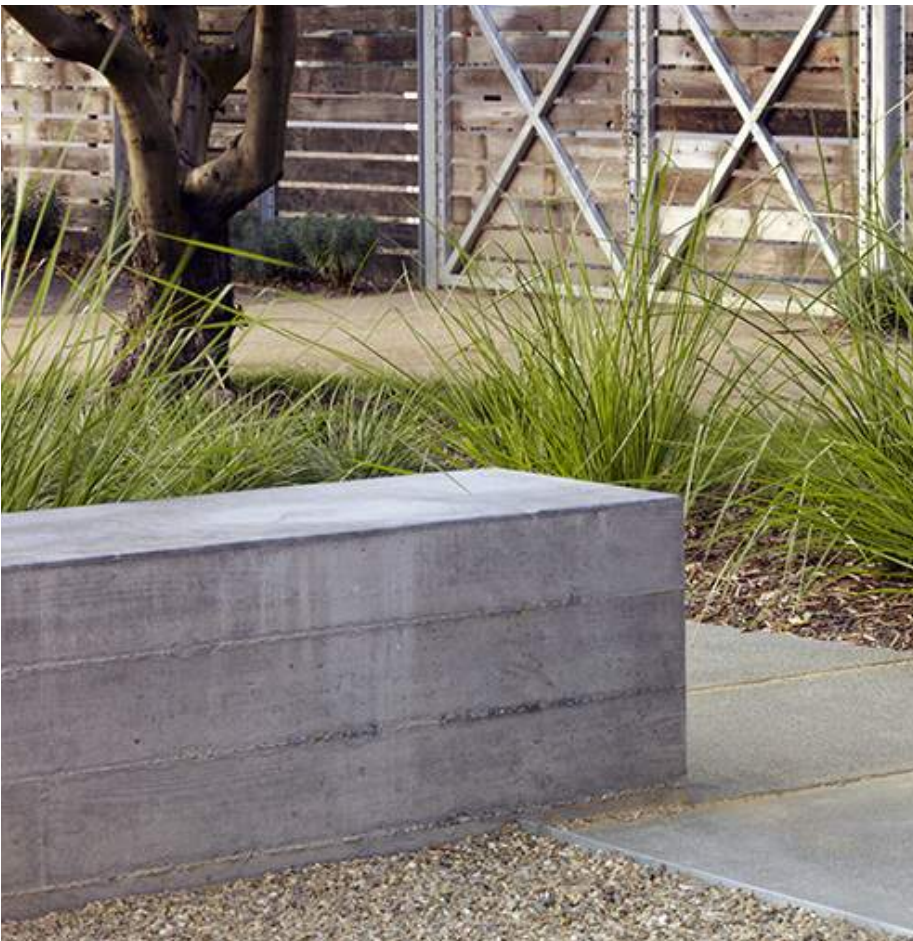
Concrete Seatwall; boardform finish Poured In Place
