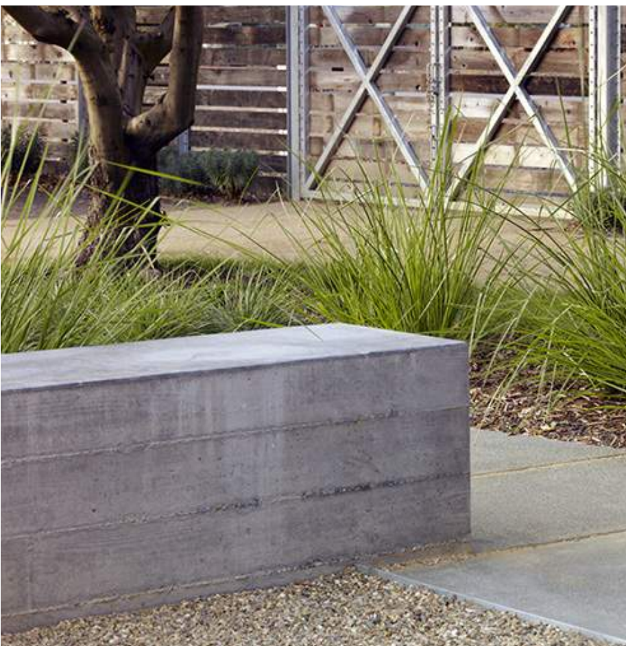
Concrete Seatwall; boardform finish Poured In Place
