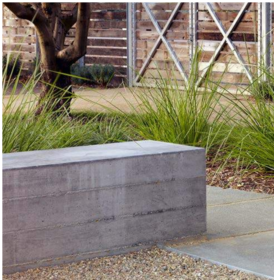
Concrete Seatwall; boardform finish Poured In Place
