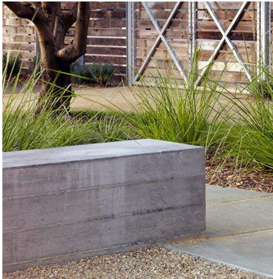
Concrete Seatwall; boardform finish Poured In Place
