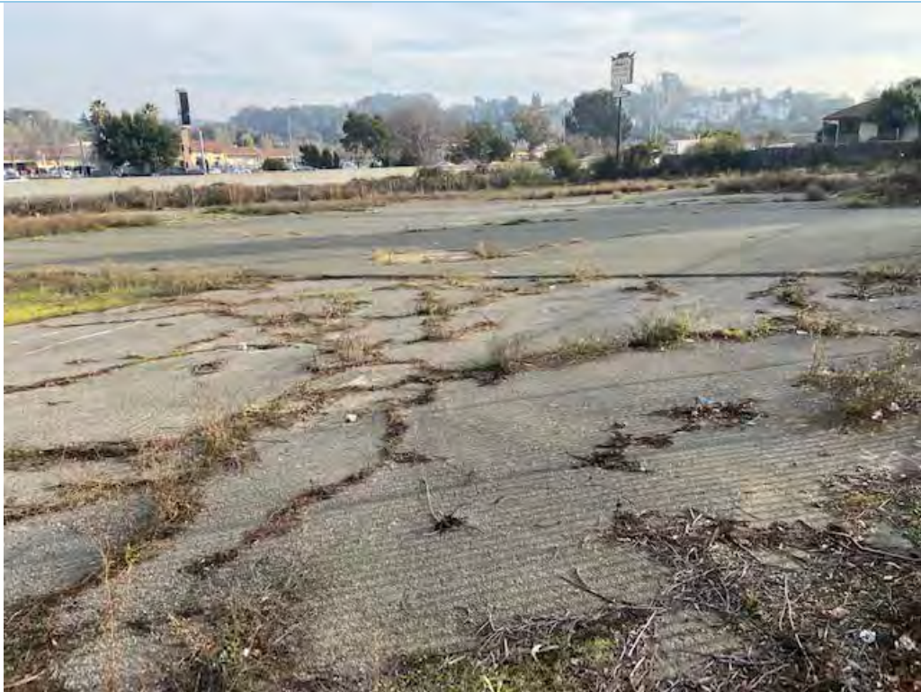
Photograph 2: View of project area; facing southeast.
