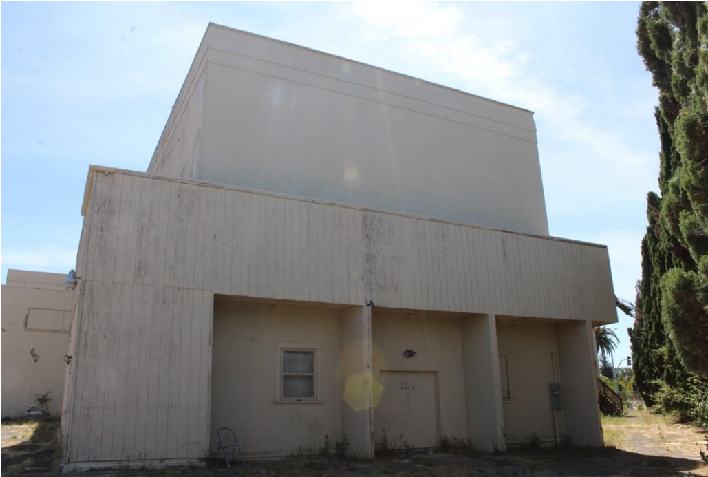
Photograph 5: West elevation of back wing, camera facing east, July 18, 2019.
