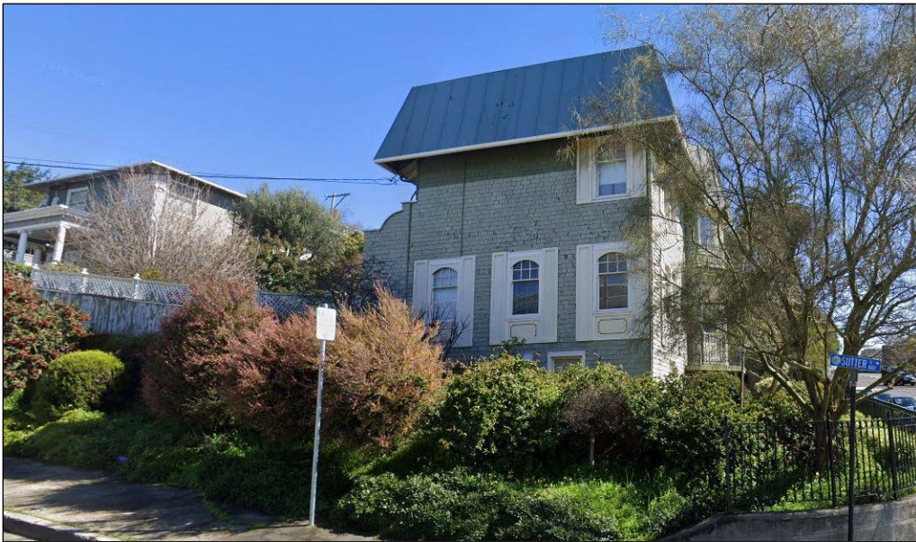
Figure 4 – Existing House (Sutter Street façade)
