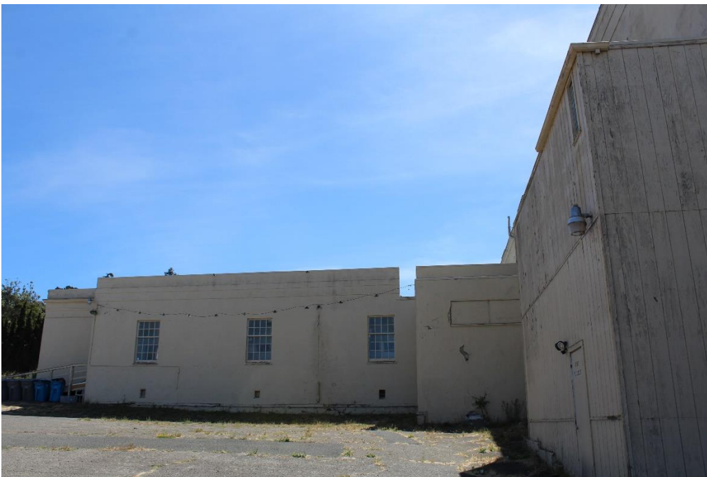
Photograph 6: West elevation and north elevation of back wing, camera facing east, July 18, 2019.
