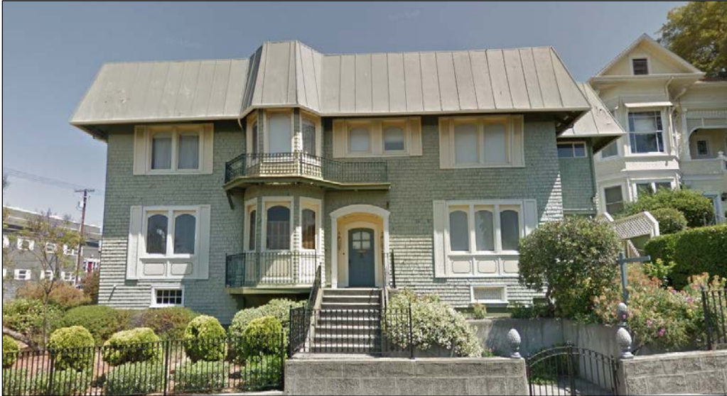
Figure 3 – Existing House (Georgia Street façade)
