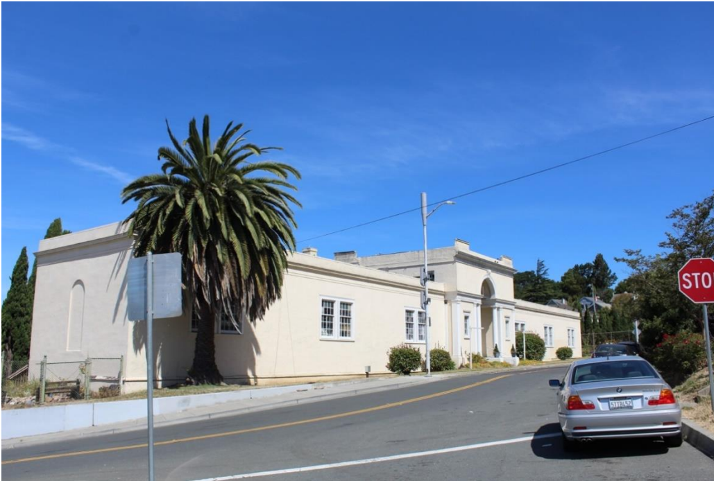
Photograph 3: South and east elevations, camera facing northwest, July 18, 2019.
