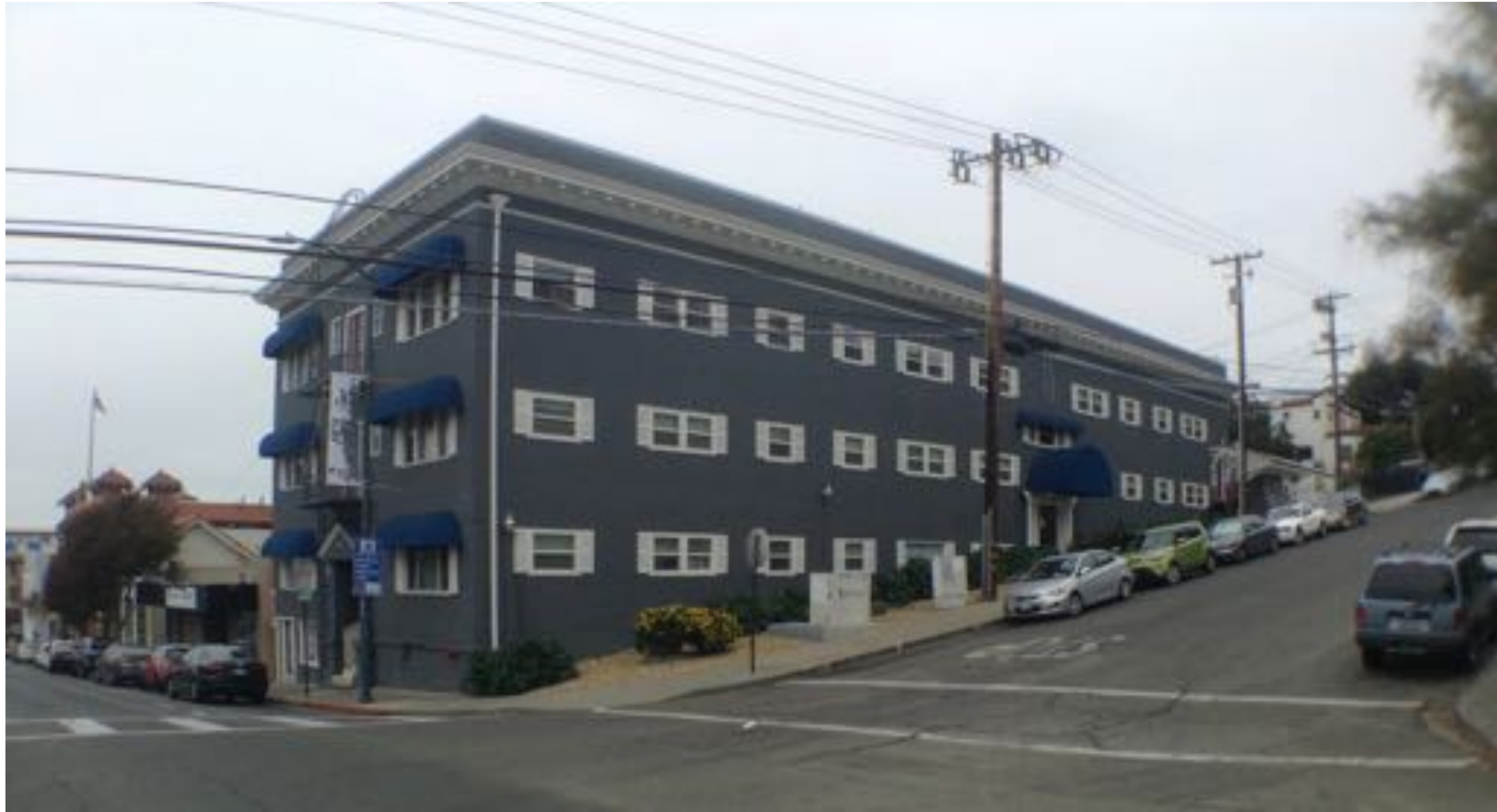
3 807 Sutter A0.3 Across Sutter street, this 3-story apartment building has a simple stucco facade but remains imposing due to its size.
