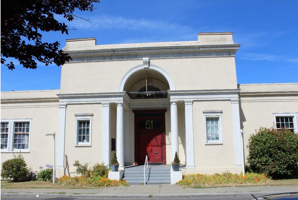
Photograph 2: Detail, main entrance, east elevation, camera facing west, July 18, 2019.
