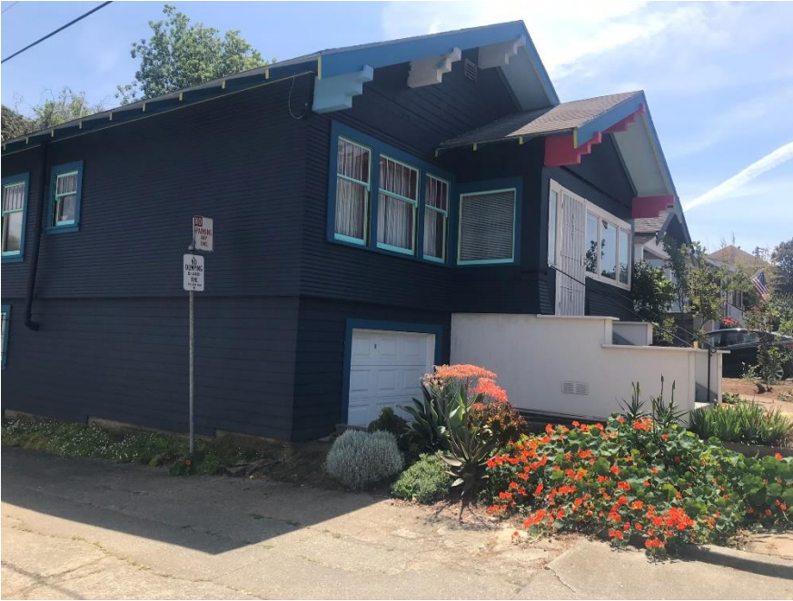
Photograph 2: North and west elevations, camera facing southeast, May 7, 2020.
