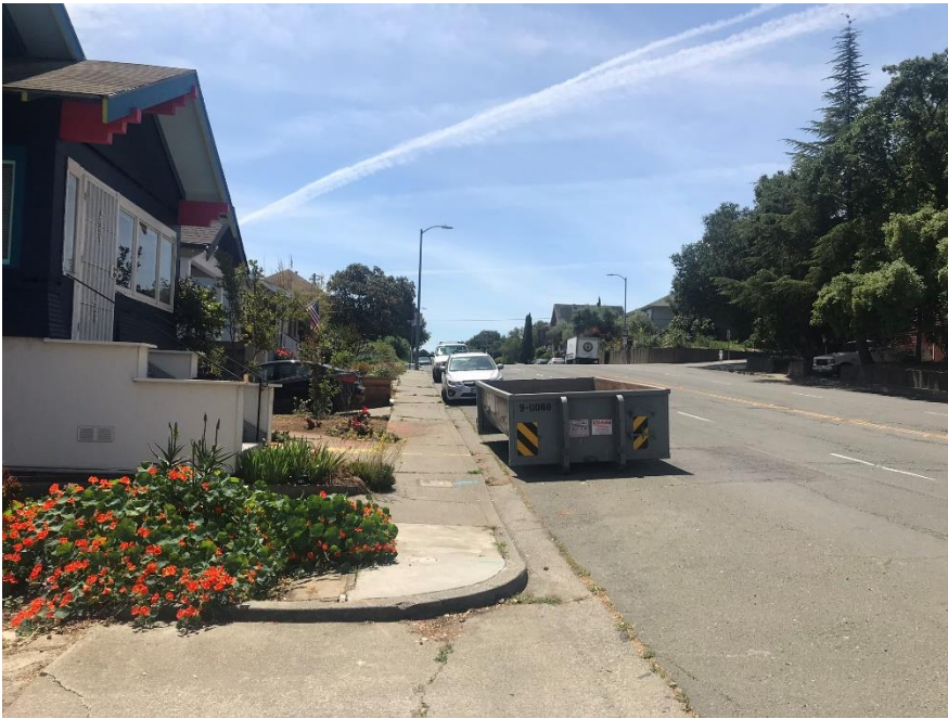
Photograph 8: View of Alameda Street at Lozier Alley, camera facing south, May 7, 2020.
