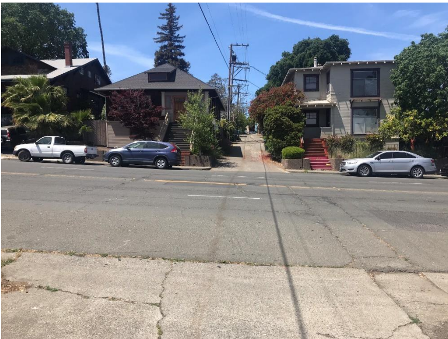
Photograph 9: View directly across from 816 Alameda Street, camera facing west, May 7, 2020.
