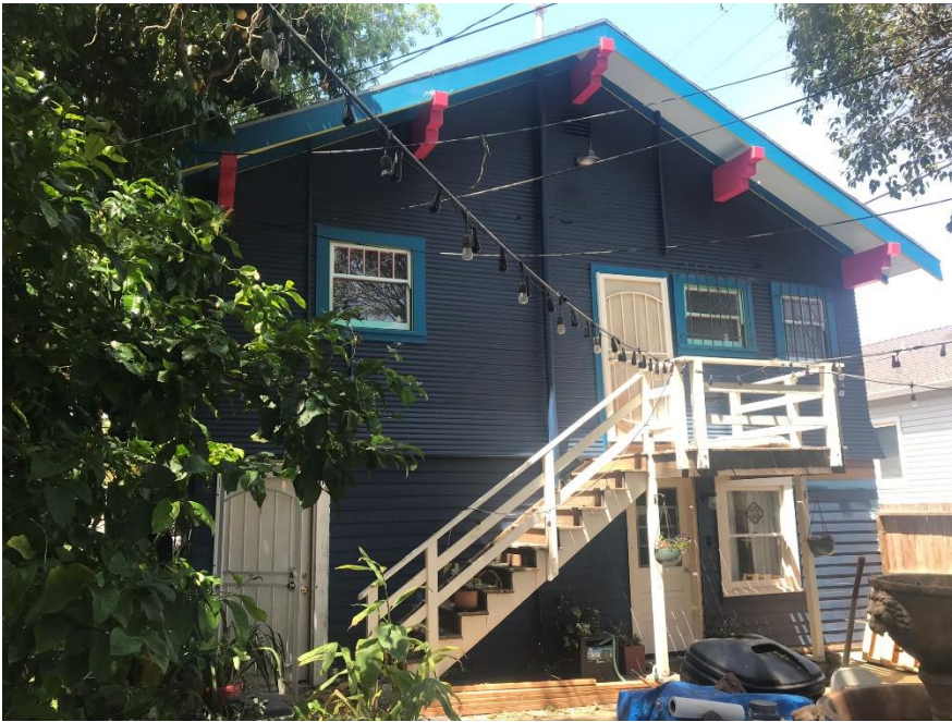
Photograph 4: East elevation, camera facing northwest, May 7, 2020.
