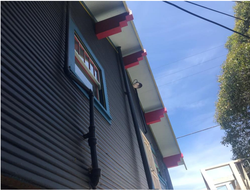
Photograph 6: Detail of rafters on eastern elevation of 816 Alameda Street, camera facing northwest, May 7, 2020.
