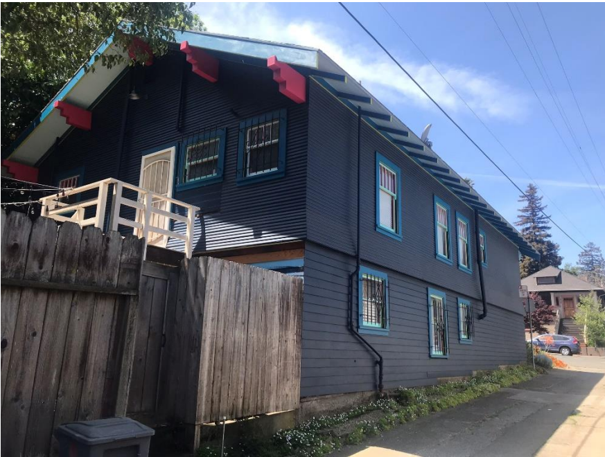
Photograph 3: North and east elevations, camera facing southwest, May 7, 2020.
