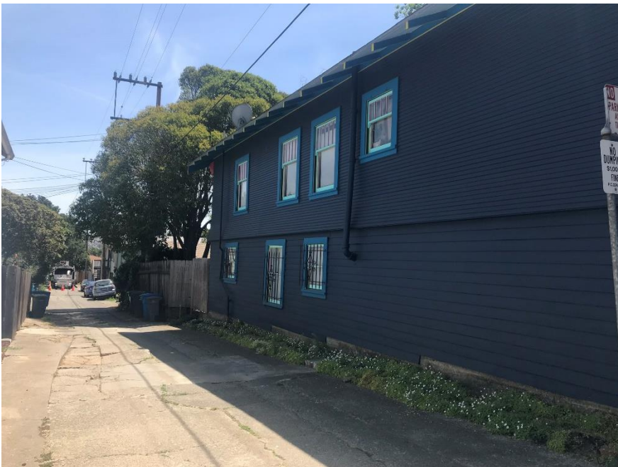
Photograph 7: North elevation of 816 Alameda Street with view of Lozier Alley, camera facing southeast, May 7, 2020.
