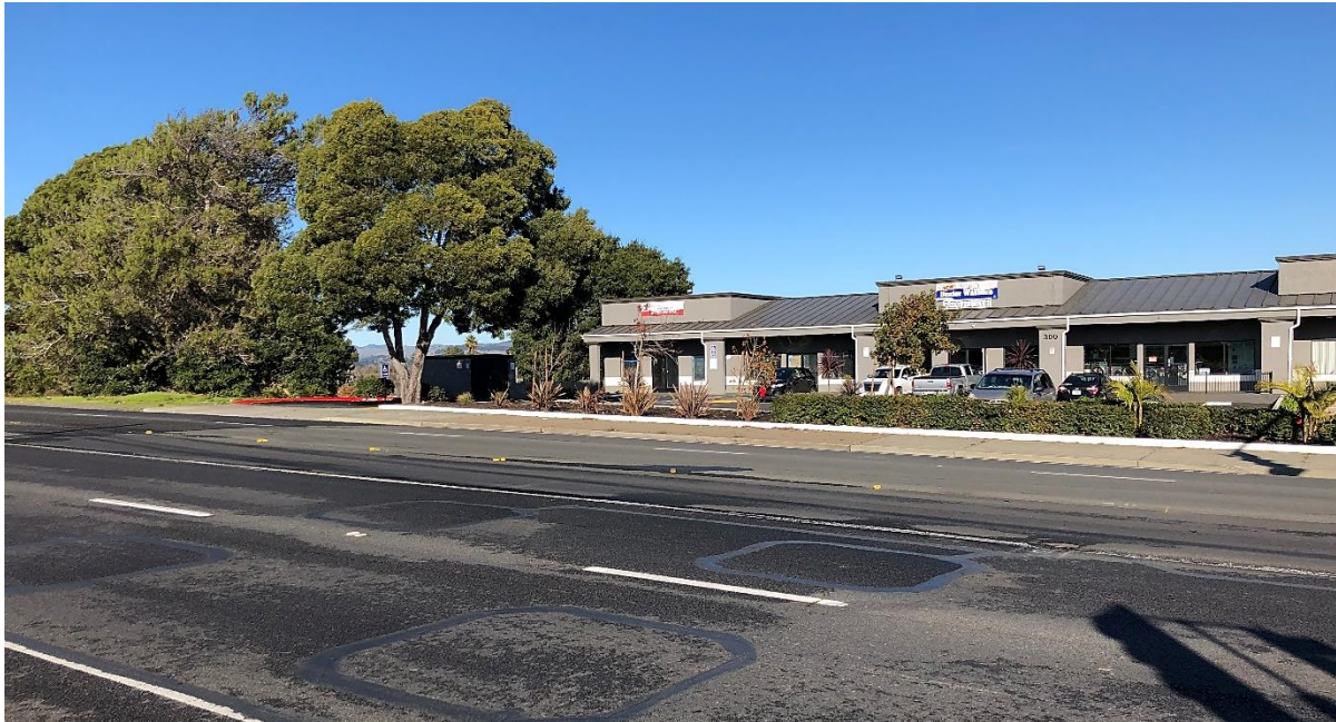
Photograph 4. View of the commercial building at the northern corner of Sonoma Boulevard and Magazine Street, facing northeast.
