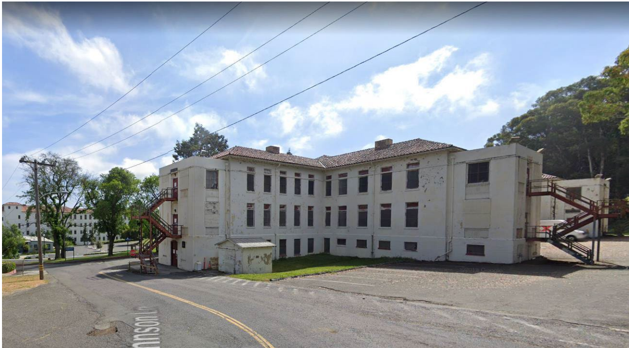
Figure 2- Photo of Building from Google Photos – with exterior staircases
