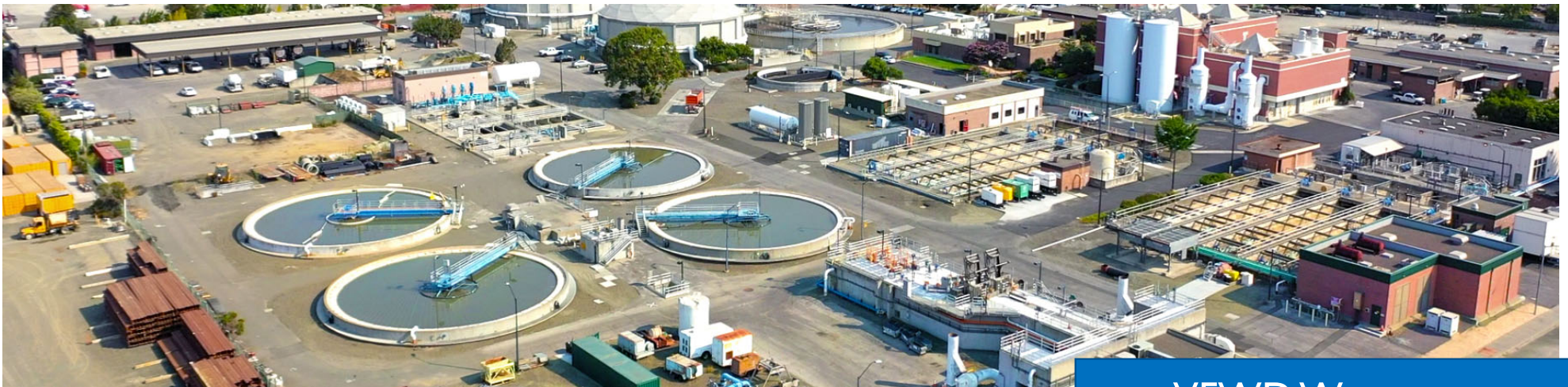
VFWD Wastewater Treatment Plant
