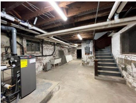
Figure 19. View of the south end of the basement.
