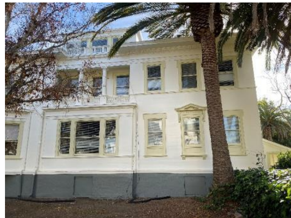
Figure 11. The rear (west) end of the northwest facade, view southeast. Courtesy of Mare Island Co.
