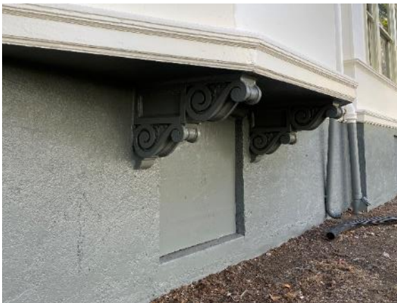
Figure 10. Scrolled brackets below the bay window, view south. Courtesy of Mare Island Co.
