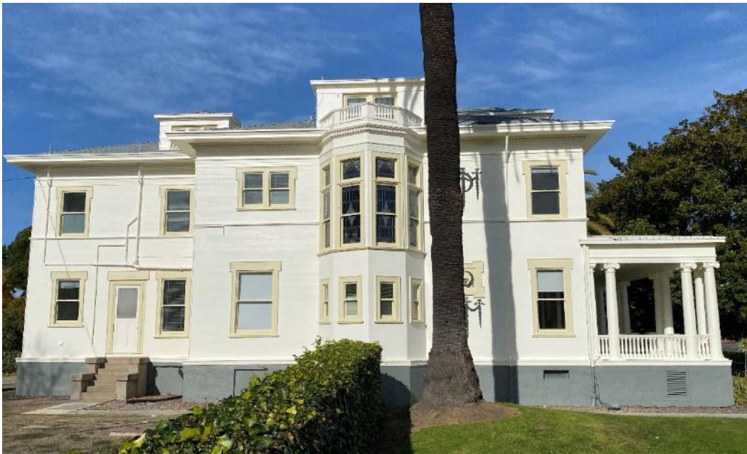
Figure 7. The southeast façade, view northwest. Courtesy of Mare Island Co.
