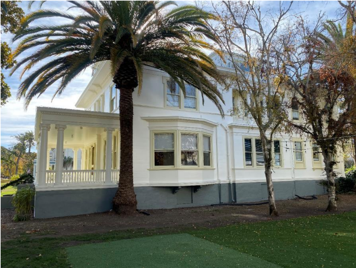
Figure 9. The east end of the northwest facade, view south. Courtesy of Mare Island Co.
