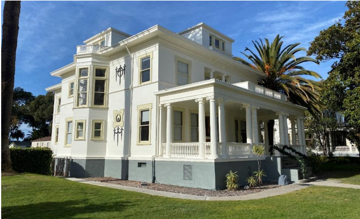
Figure 3. Officer's Quarters N, view west. Courtesy of Mare Island Co.
