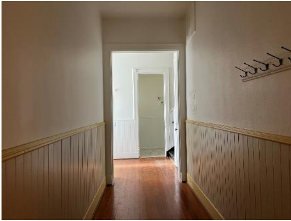
Figure 28. The first-floor corridor, view southwest.
