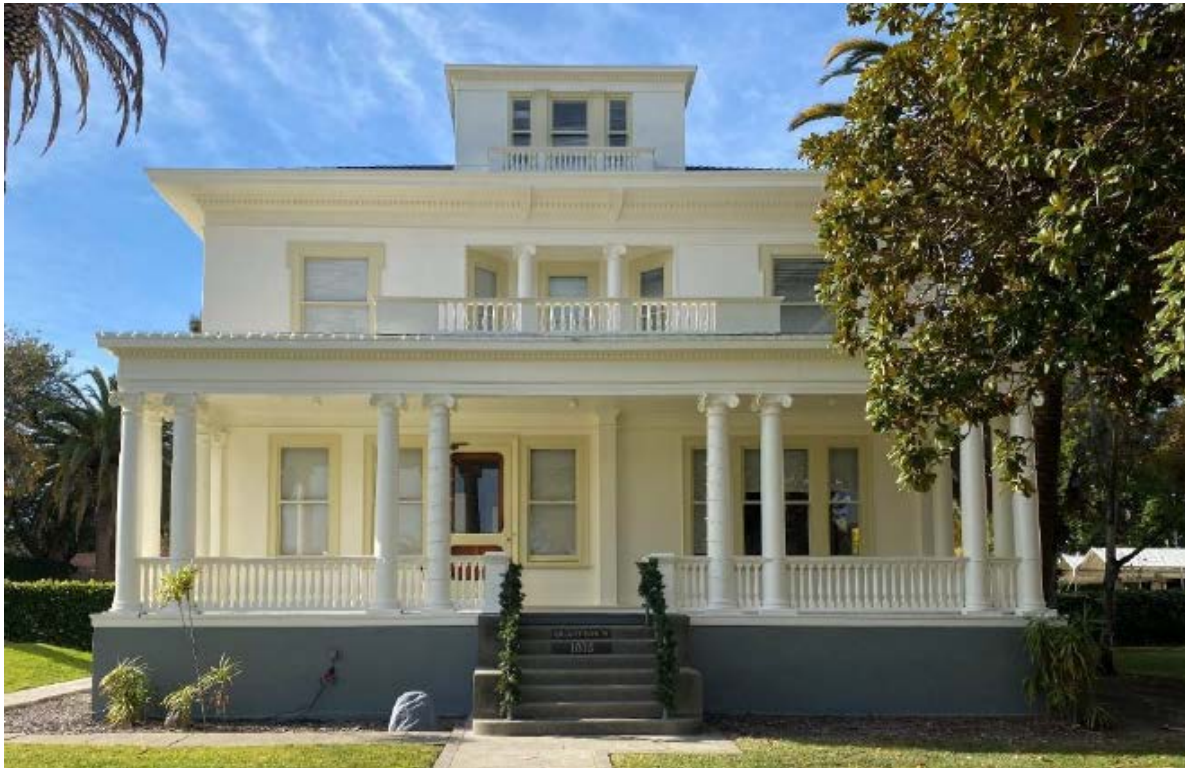
Figure 2. Officer's Quarters N (primary facade)
