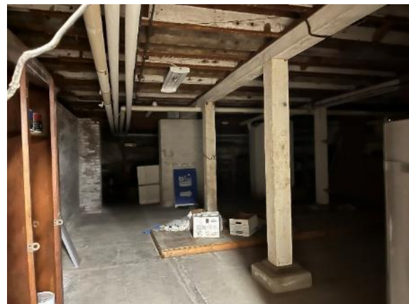
Figure 20. View of the north end of the basement.
