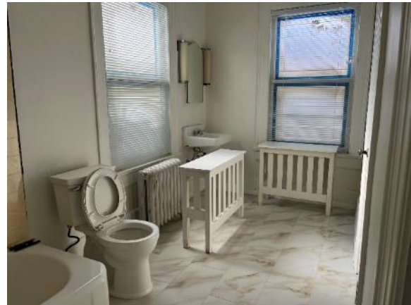
Figure 37. One of the second-floor restrooms.
