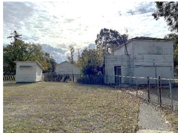
Figure 14. Building N-H and chain link fence at the rear of the property, view southeast.
