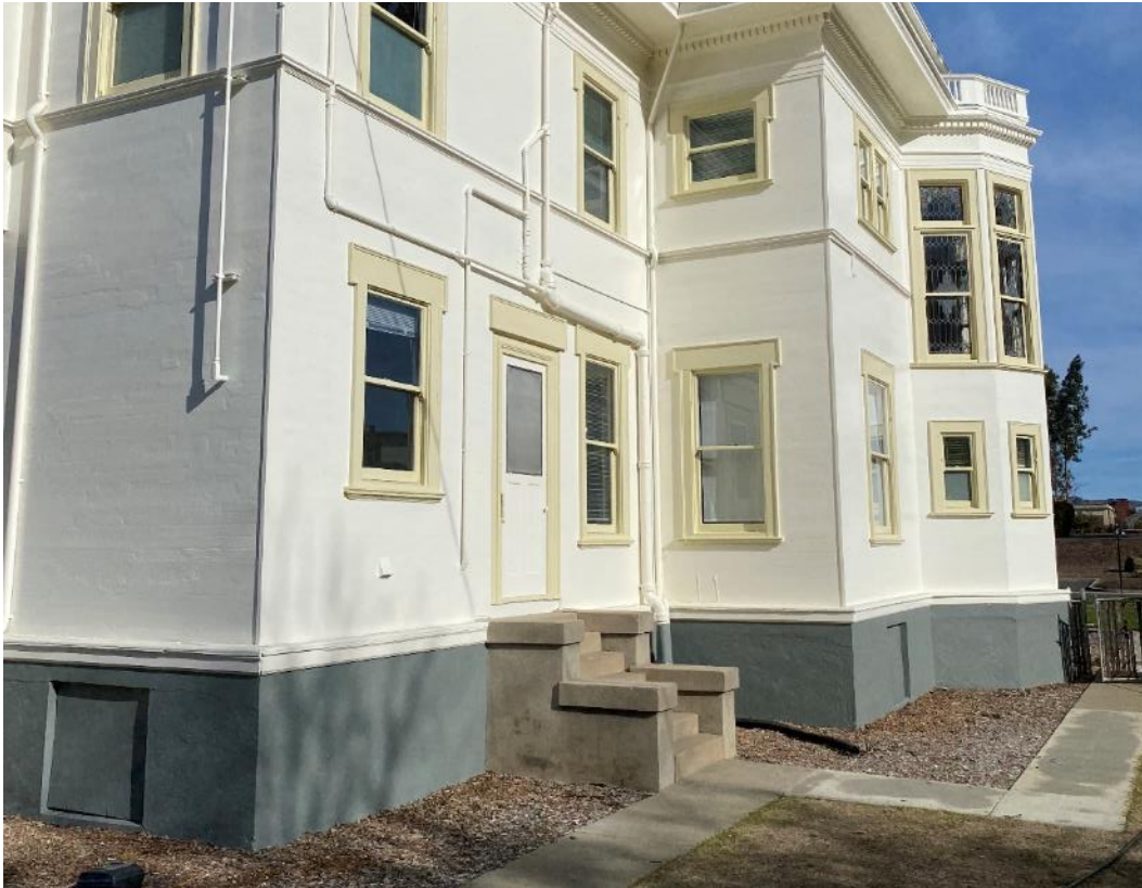
Figure 8. The recessed portion of the southeast façade, view north. Courtesy of Mare Island Co.
