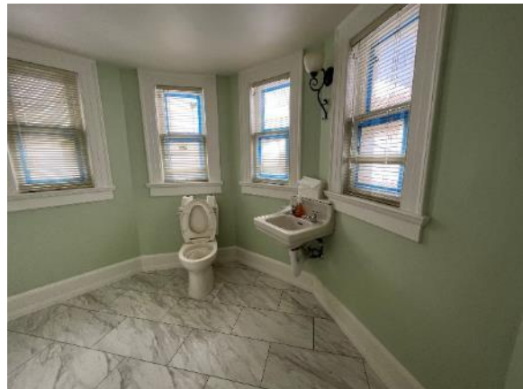
Figure 27. The first-floor restroom, view east.
