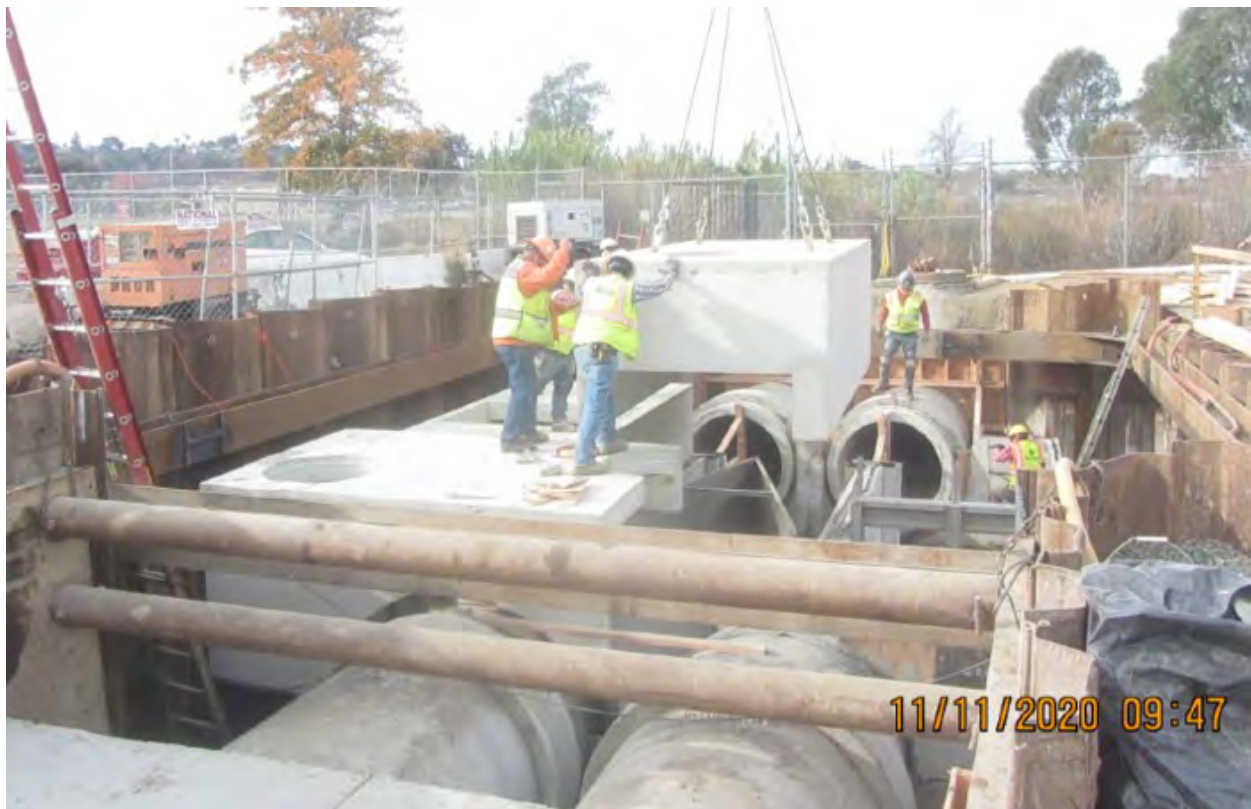
Construction of a stormwater trash capture device.
