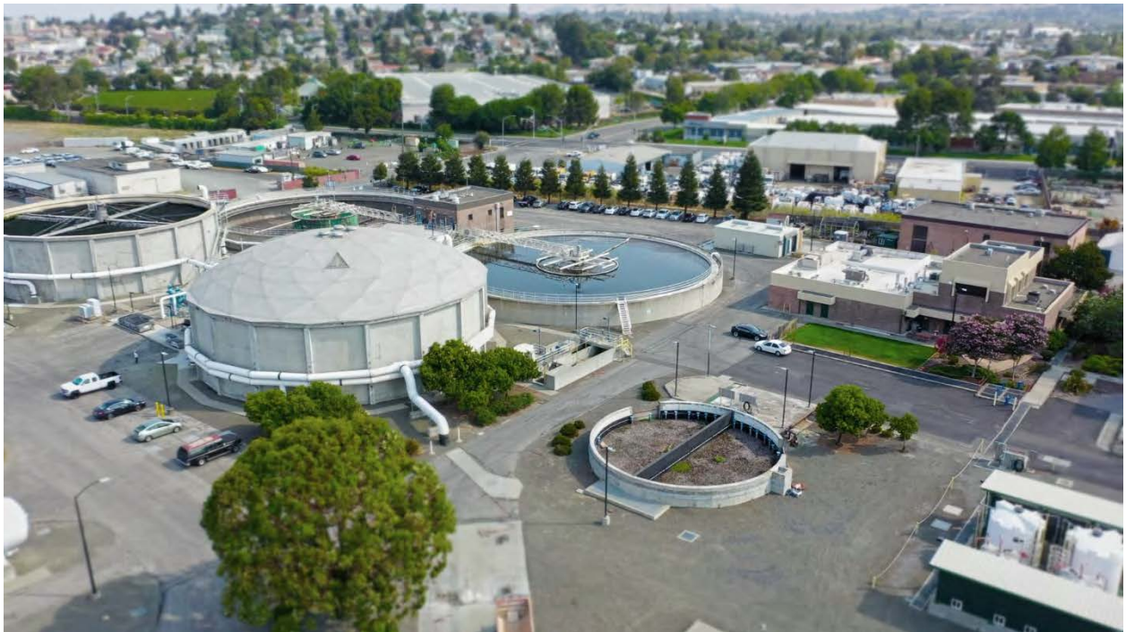
Vallejo Flood and Wastewater District treatment plant, highlighting biotower and secondary clarifier.
