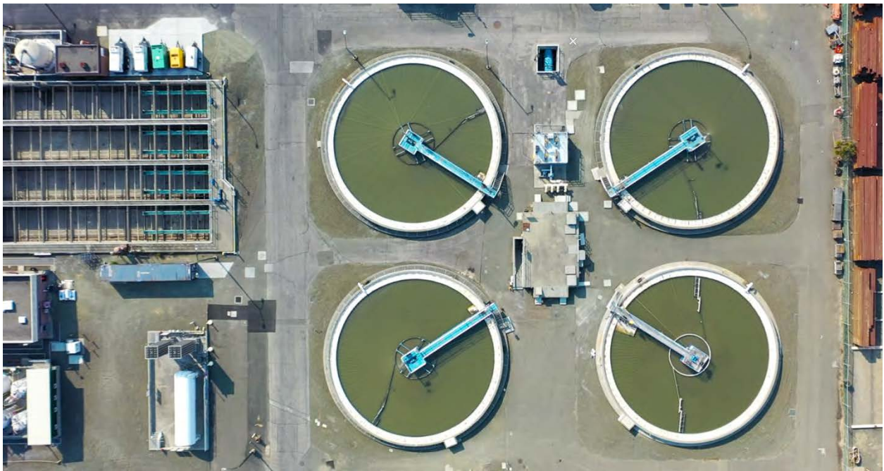
Vallejo Flood and Wastewater District treatment plant, highlighting four primary clarifiers.
