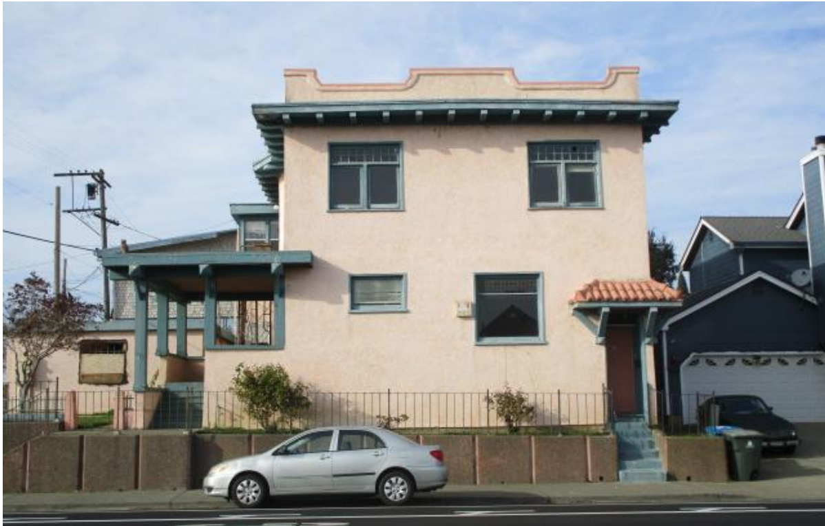
Figure 2 View of East Elevation
