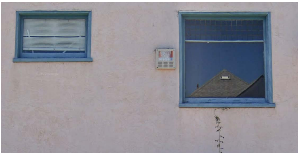
Figure 3 – Character Defining Windows
