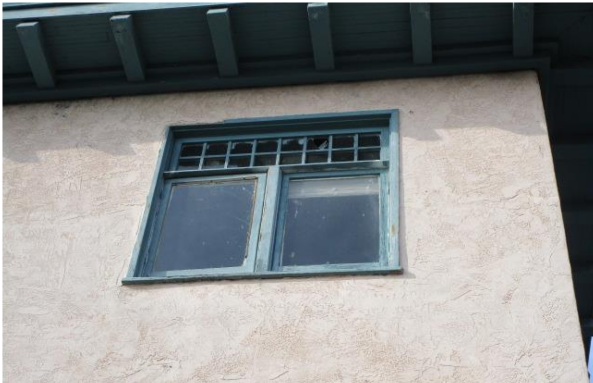
Figure 5 View of East Elevation Second Floor Casement Windows
