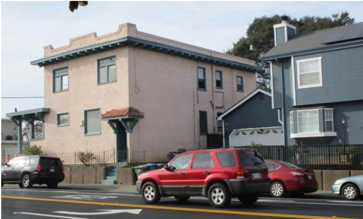
Figure 3 View of East and North Elevations
