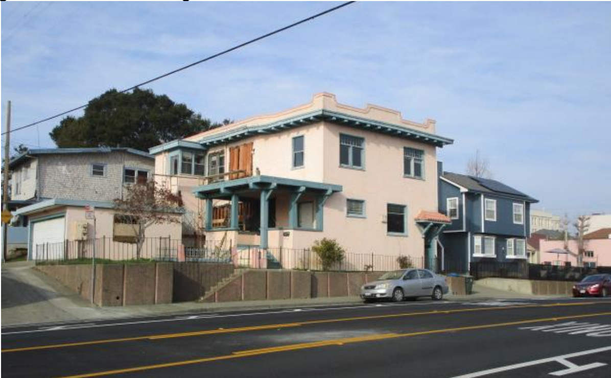
Figure 1 View of the Building's South and East Elevations
