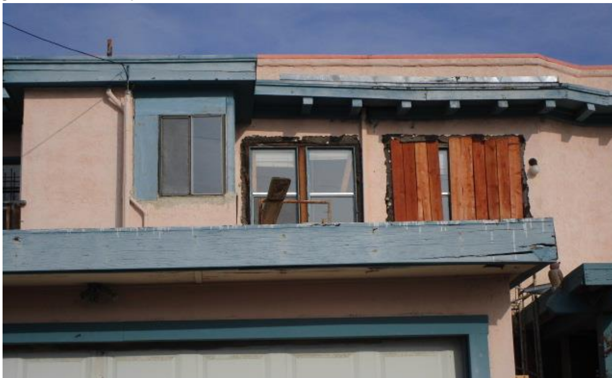
Figure 6 View of Replaced Second Floor Windows on South Elevation
