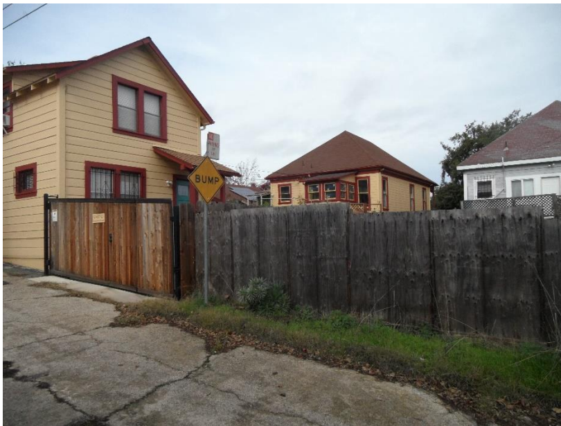
View of project east of auxiliary dwelling unit from Overland Alley.
