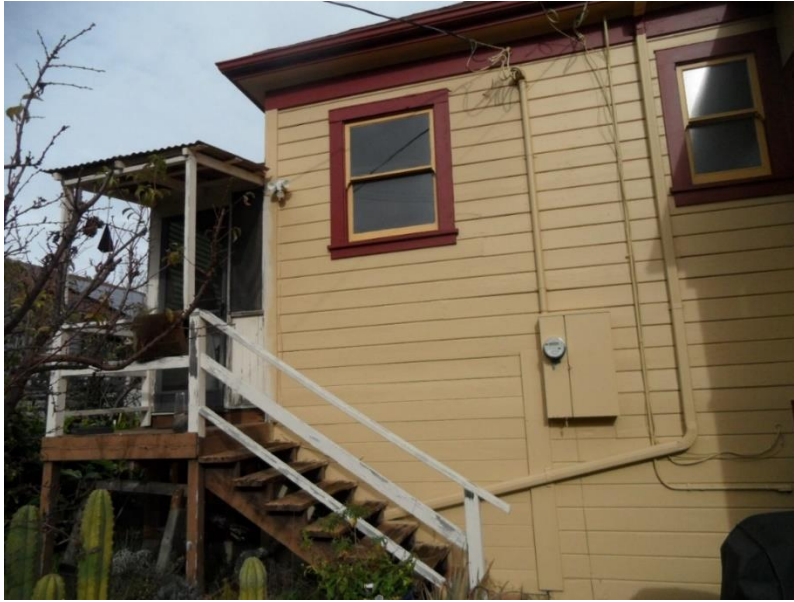
Closeup of existing corrugated fiberglass awning, landing, and stairs.
