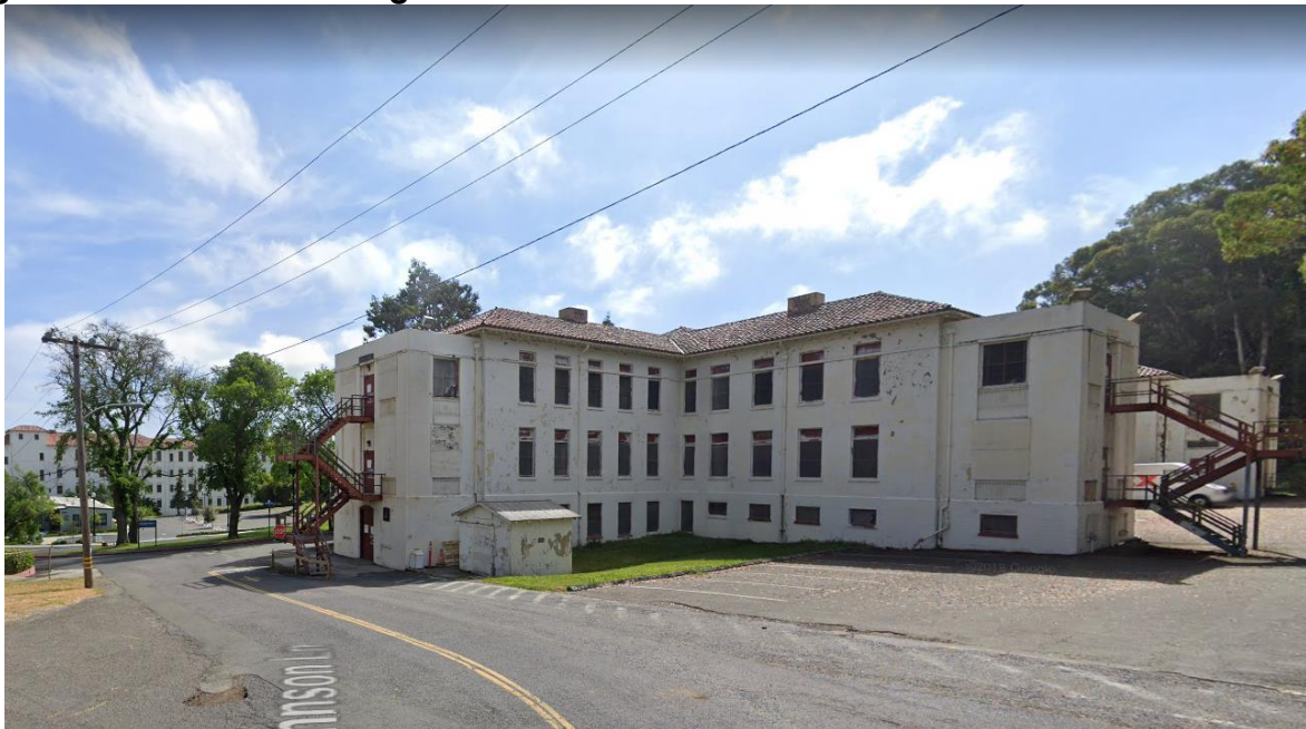
Figure 1 View of the Building’s South and West Elevations Prior to Stair Removal
