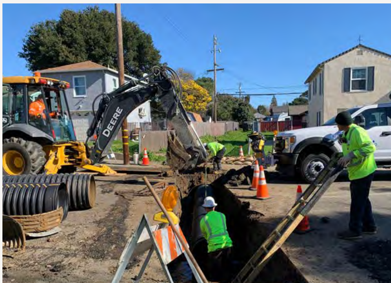
Repairs being made on Hermosa Avenue
