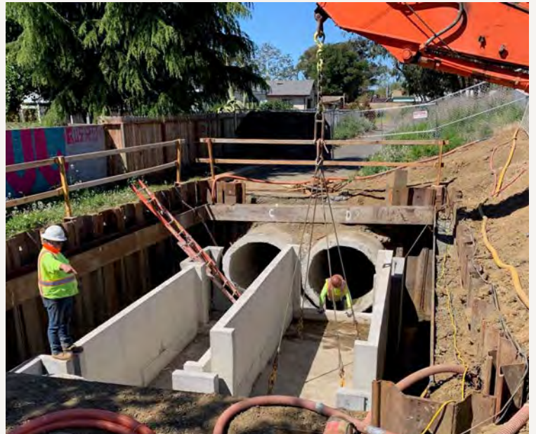
Construction is underway on this stormwater trash capture device
