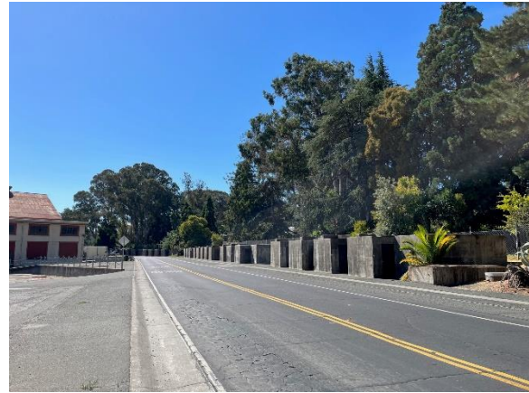
Figure 5. Row of concrete bomb shelters along Railroad Avenue, view south.
