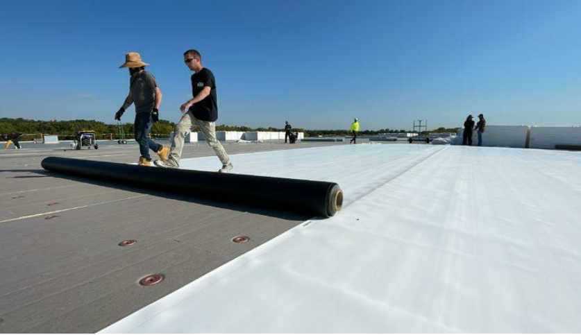
TPO ROOF MEMBRANE
