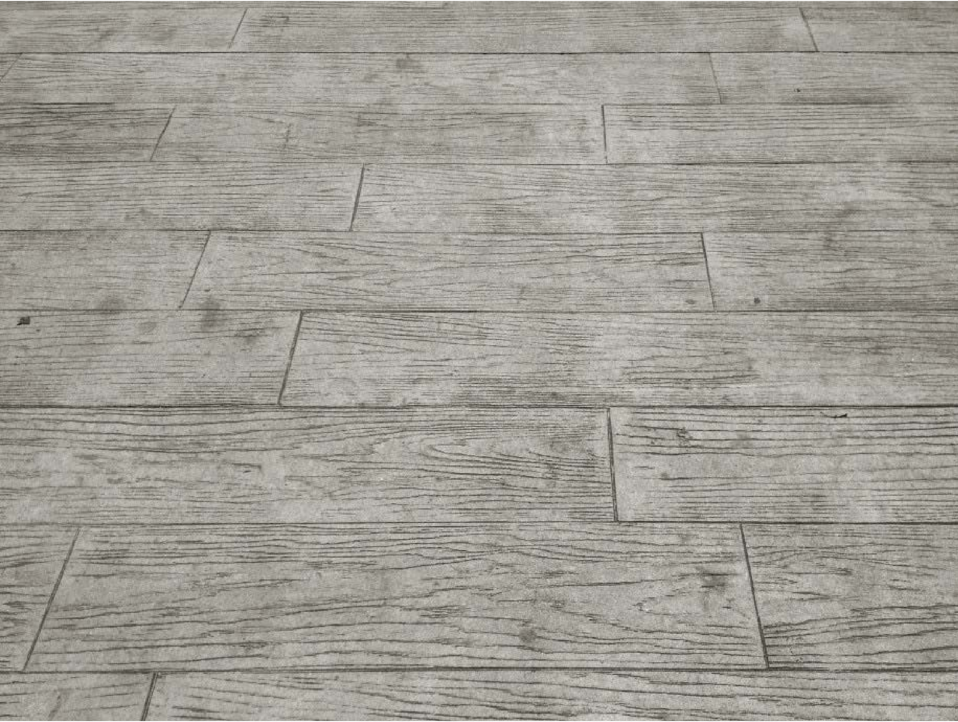
Stamped 'board' concrete paving
