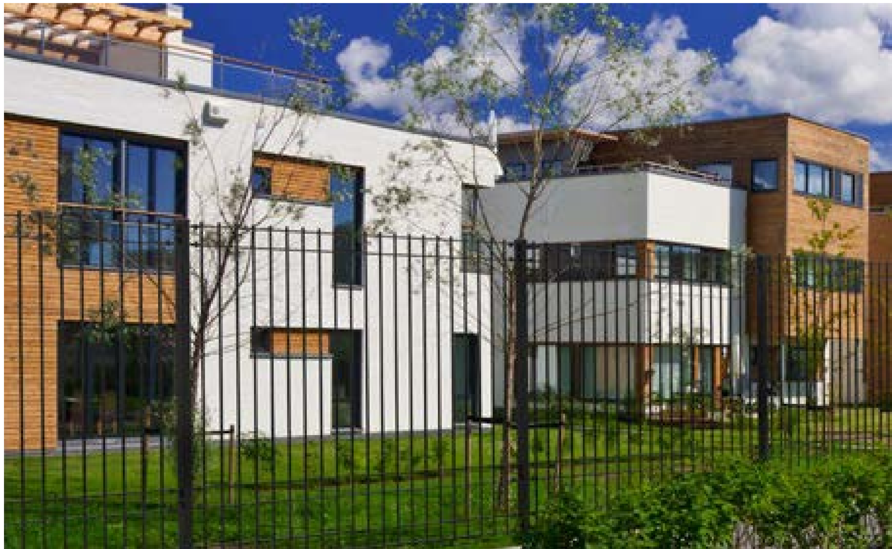
Metal residential security fence
