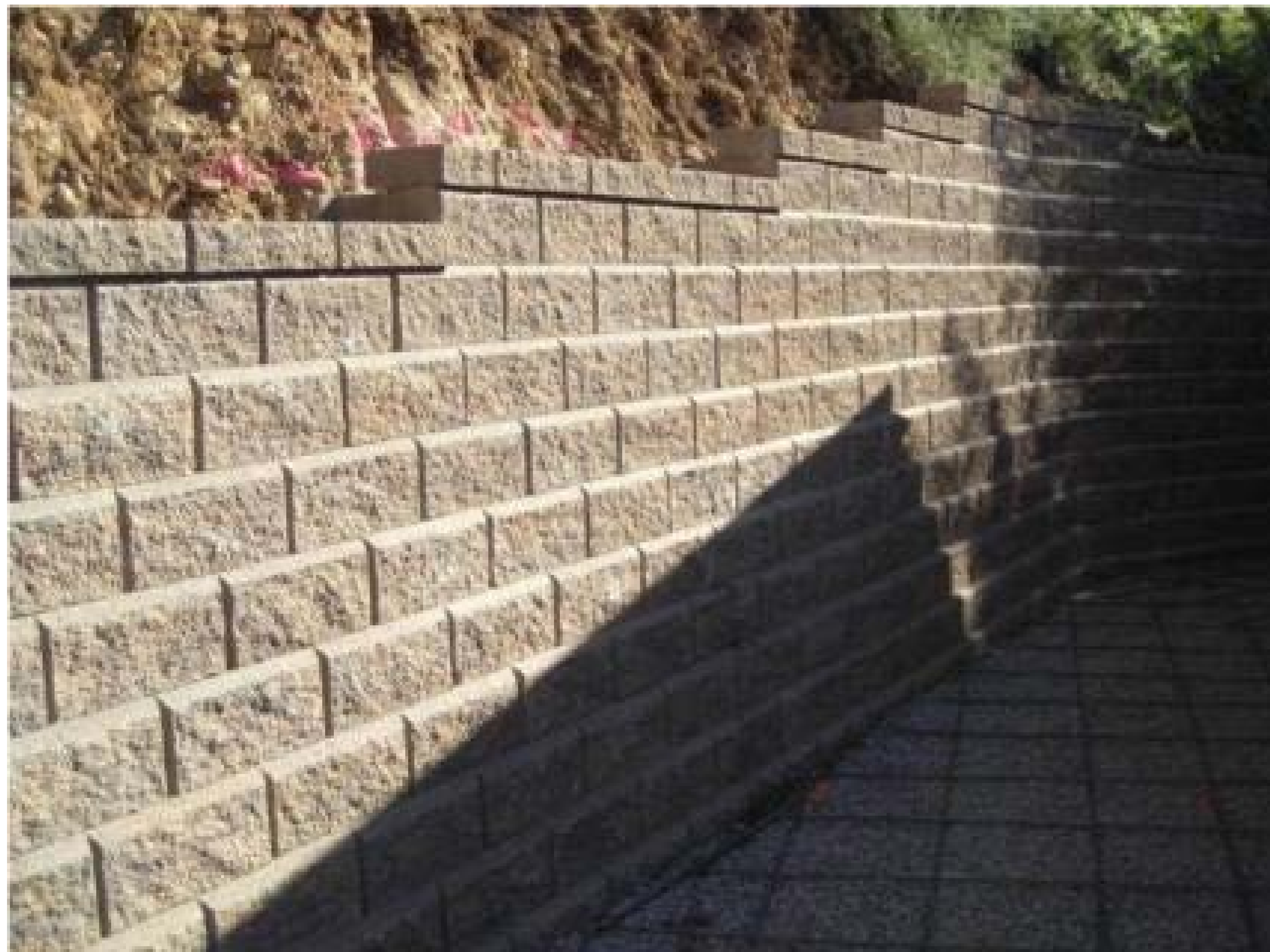
Block retaining wall
