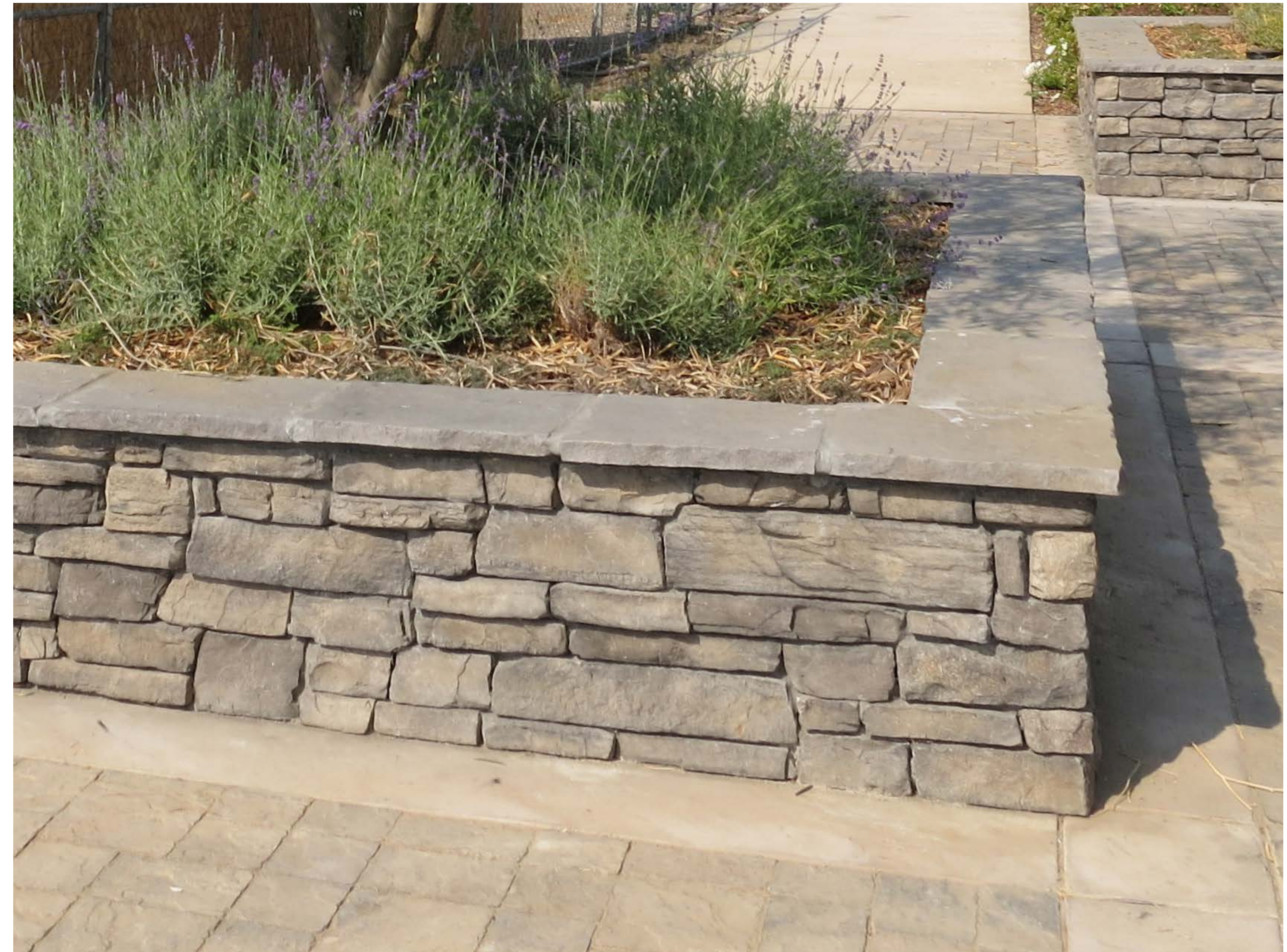
Stone-clad planter wall
