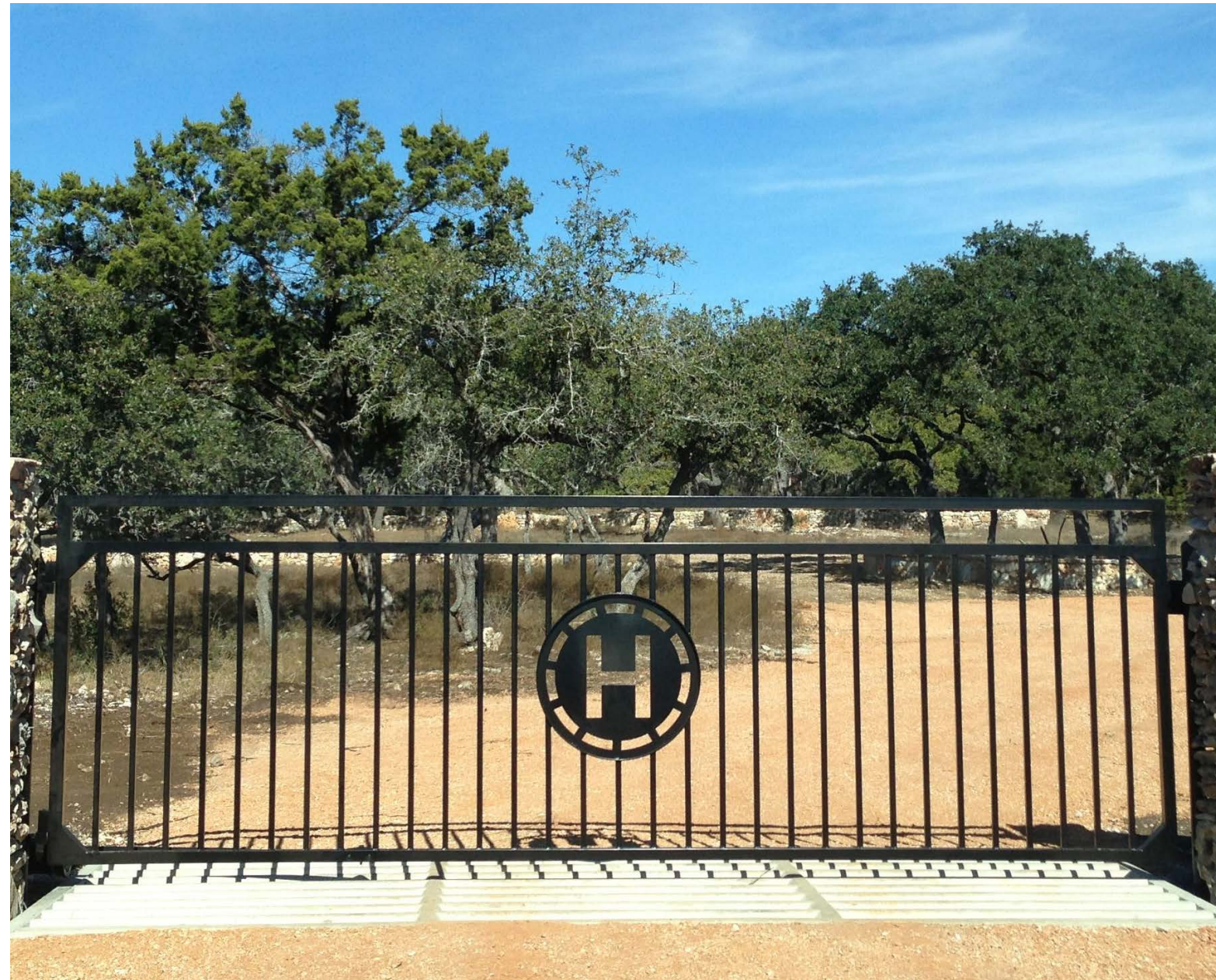
Security gate with pilasters (w/ Knox Box)
