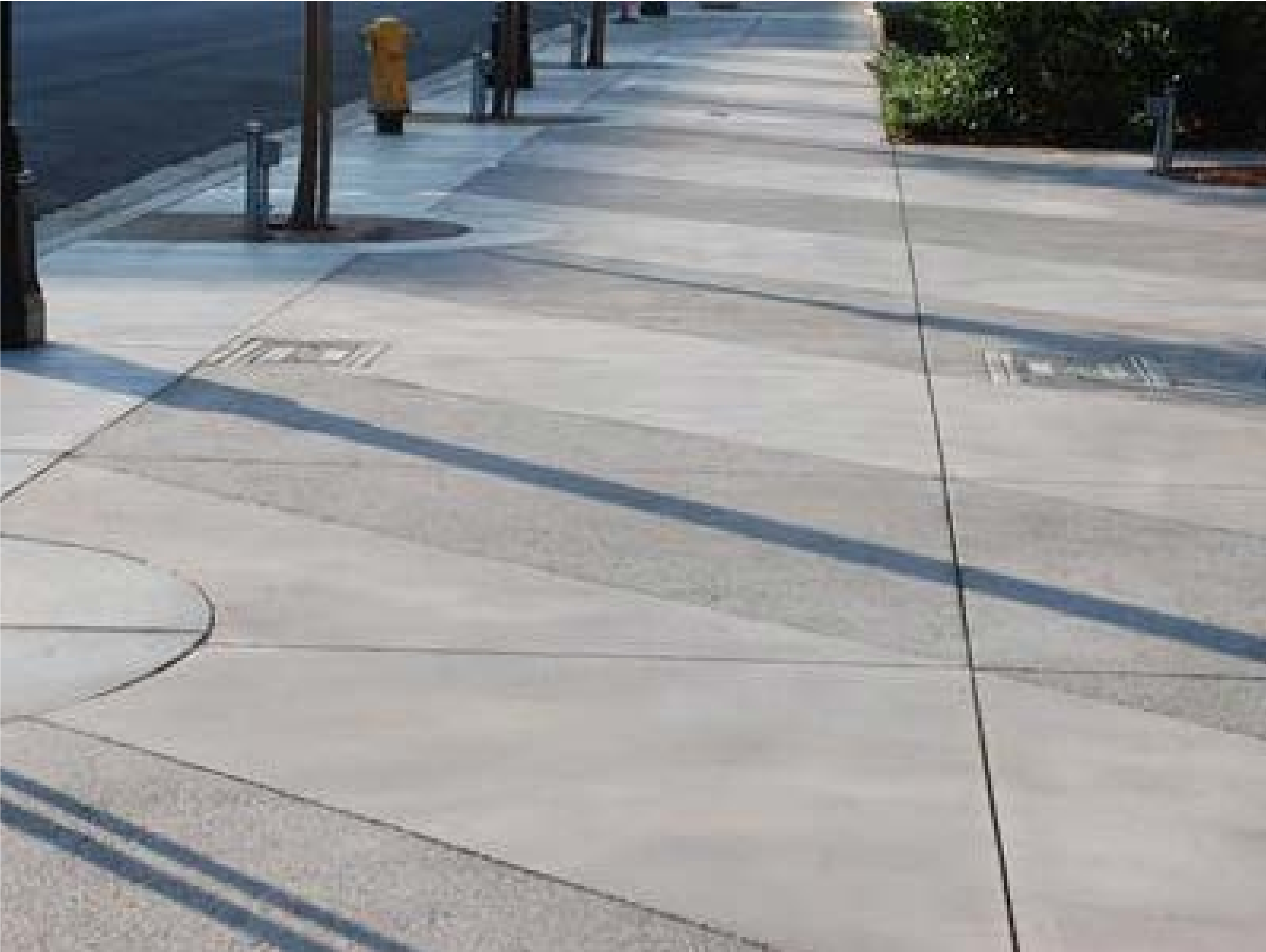
'Acid etch' concrete paving
