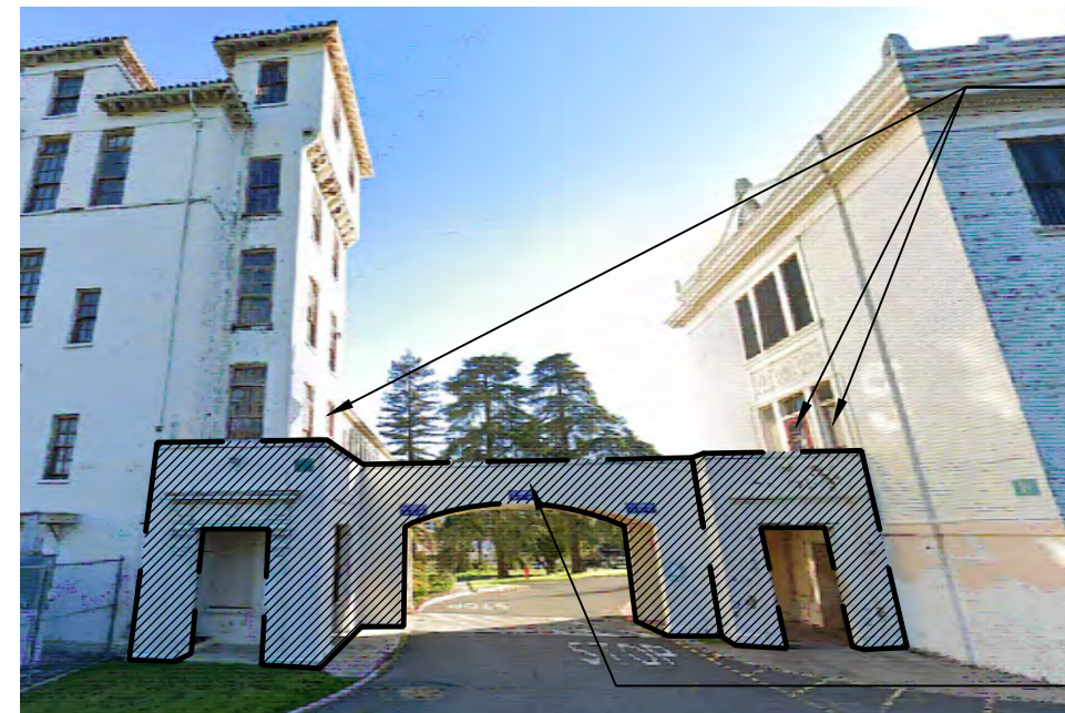
4 SOUTH WEST WING BRIDGE SOUTH WEST VIEW
