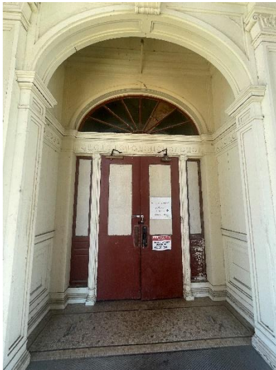
Figure 4. The entry vestibule, view southwest.
