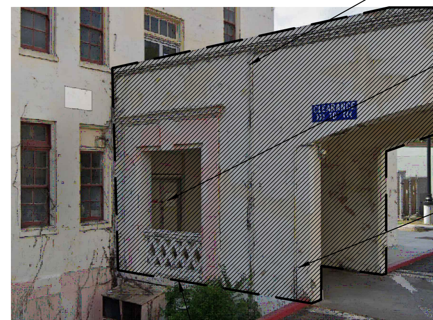
7 H1 SOUTH EAST WING NORTH EAST VIEW
