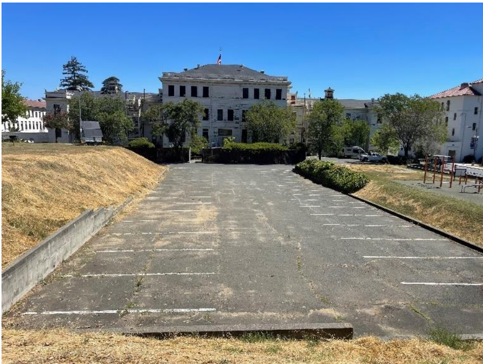
Figure 14. The rear of the building, view northwest.
