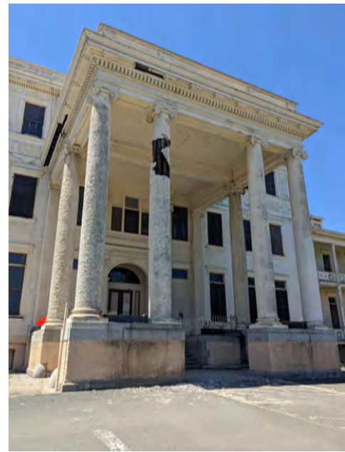
PORTE COCHERE WILL BE RECONSTRUCTED TO MATCH ORIGINAL CONDITION
