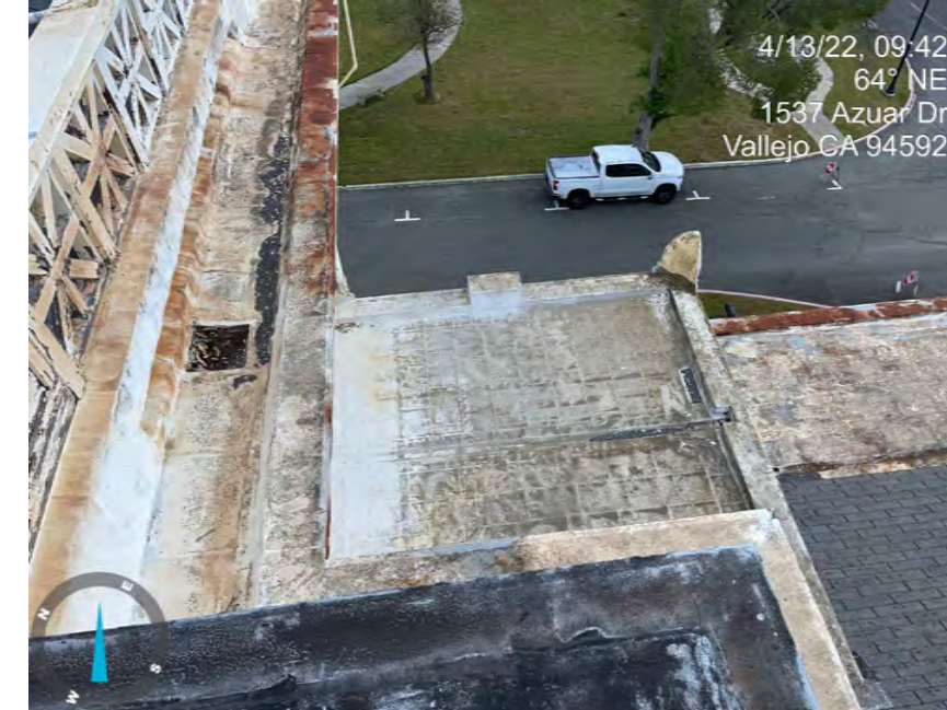
EXISTING ROOF DRAIN, CONCEALED GUTTER EDGE AT LOWER FLAT ROOF. SEE SHEET NOTES FOR SCOPE OF WORK INFORMATION
