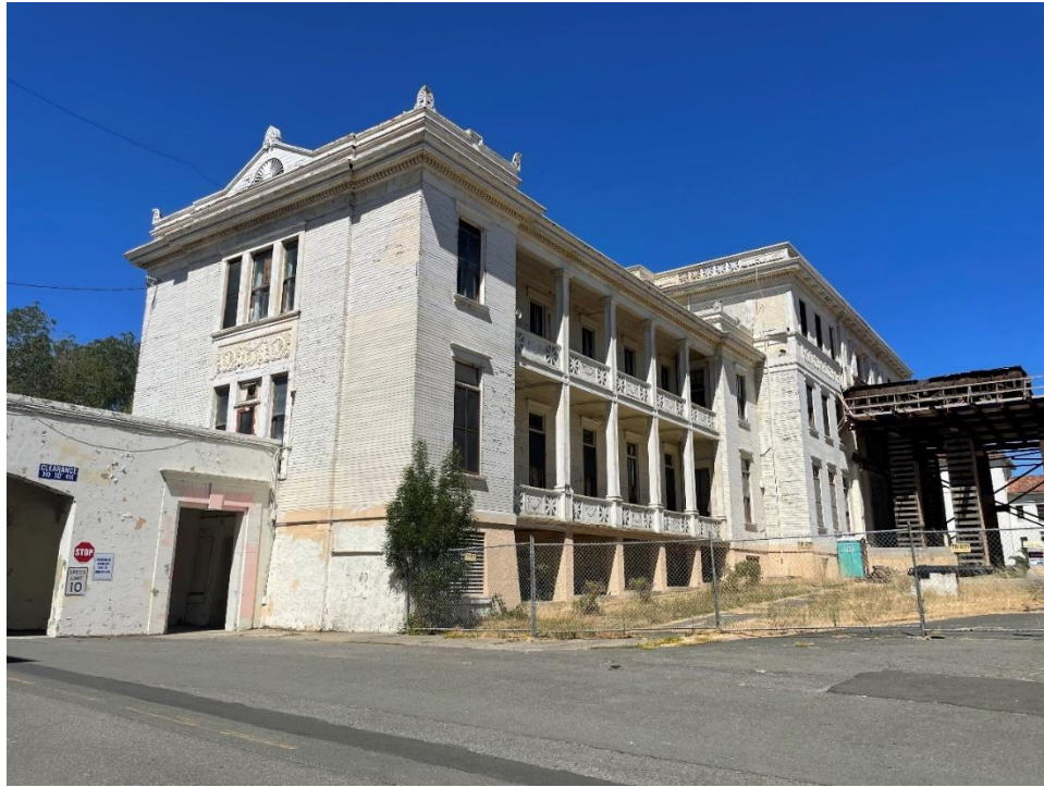
Figure 6. Oblique view of southeast face, view west.
