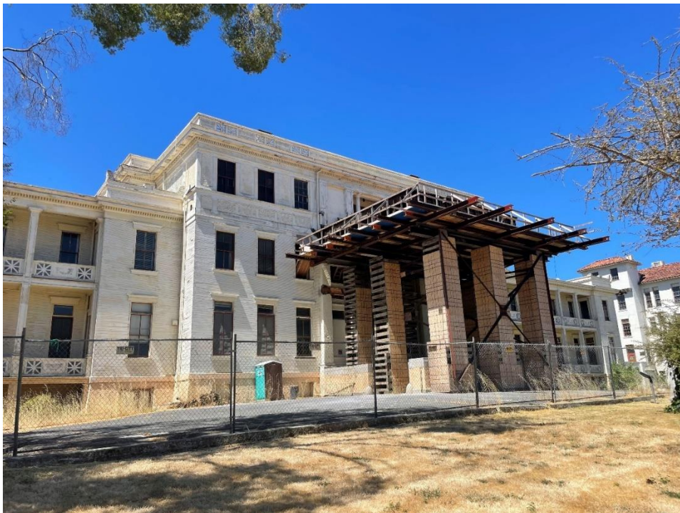
Figure 3. Primary (northeast) façade porte-cochère, view west.
