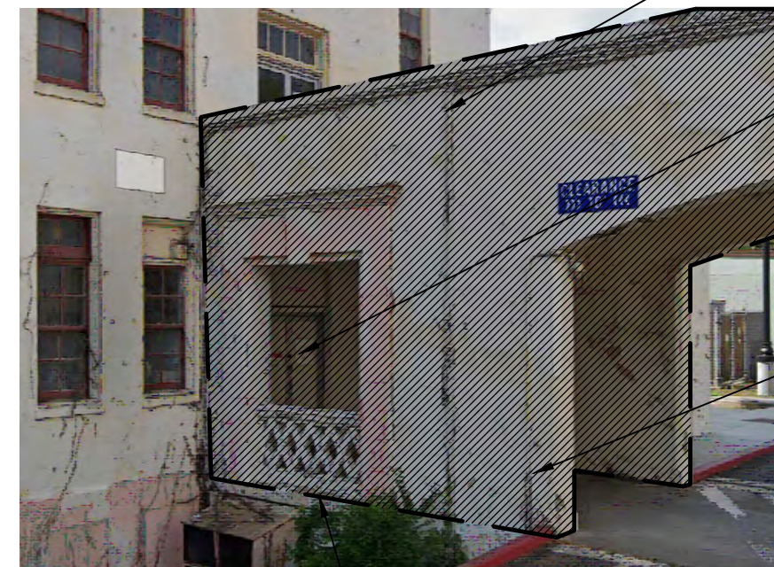
7 H1 SOUTH EAST WING NORTH EAST VIEW
