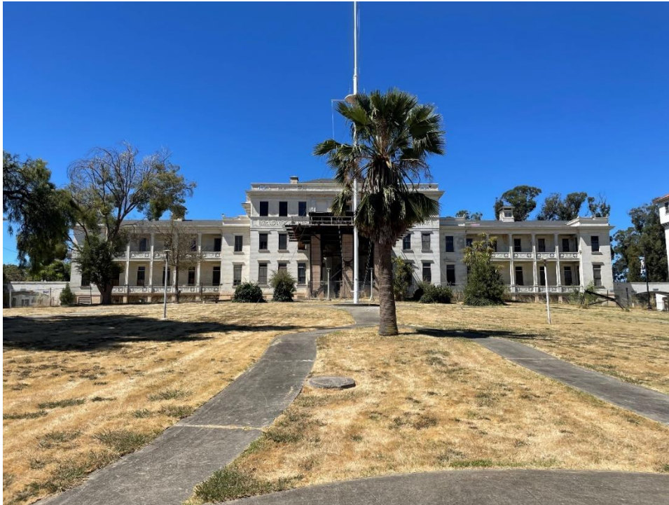
Figure 2. Building H1, view southwest.
