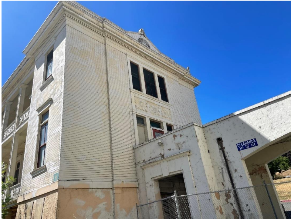
Figure 12. Oblique view of northwest façade and connecting arch, view south.
