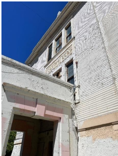
Figure 7. Detailed view of southeast façade and connecting arch, view west.
