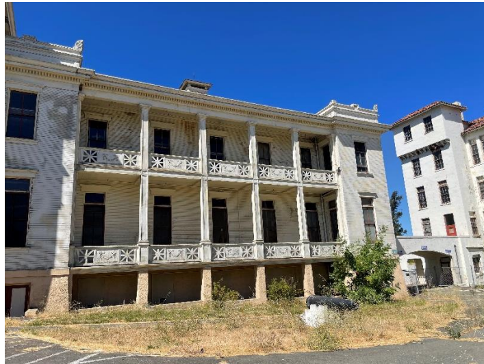
Figure 5. The colonnaded veranda with pavilion, view west.
