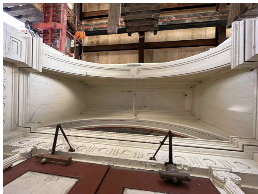
ORNAMENTAL MOLDING, TRIM, AND WOOD PANELING, SEE SHEET NOTES FOR SCOPE OF WORK INFORMATION
