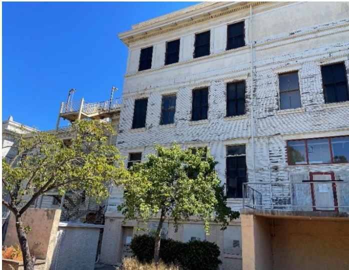
Figure 10. Central projecting section of rear (southwest) facade, view northeast.
