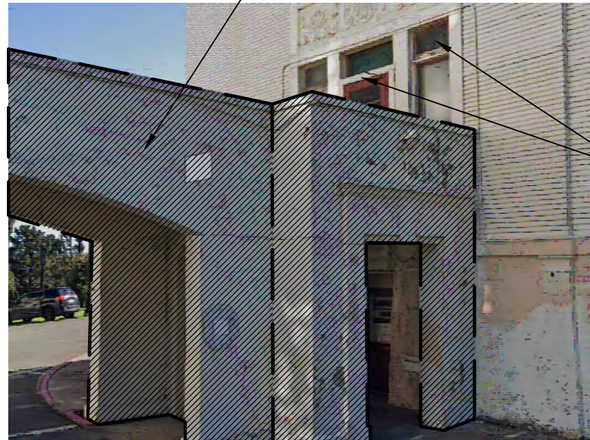
3 H1 MAIN BLDG NORTH WEST SOUTH EAST VIEW
