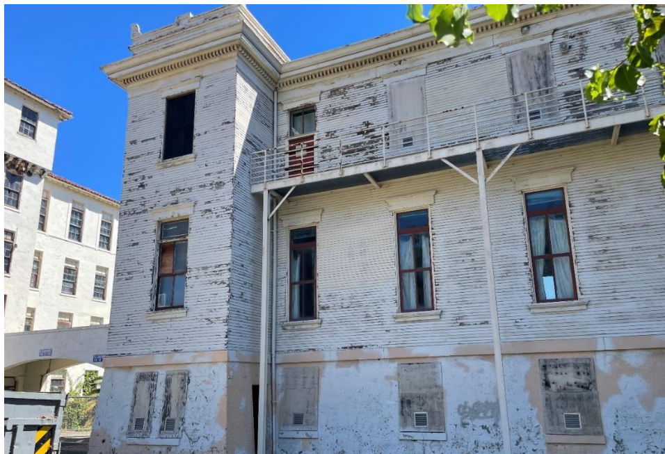
Figure 9. Rear (southwest) façade with narrow pavilion, view northeast.
