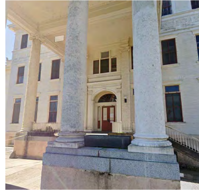
ALL FRONT FACADE AREAS EFFECTED BY PORTE COCHERE RECONSTRUCTION TO BE REPAIRED AND RESTORED TO MATCH ORIGINAL CONDITION.
