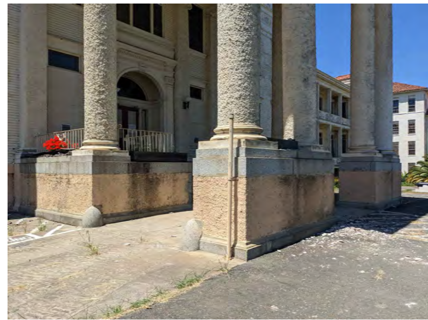
GRANITE AND PLASTER BASE WILL BE CLEANED AND RESTORED TO MATCH ORIGINAL CONDITION
