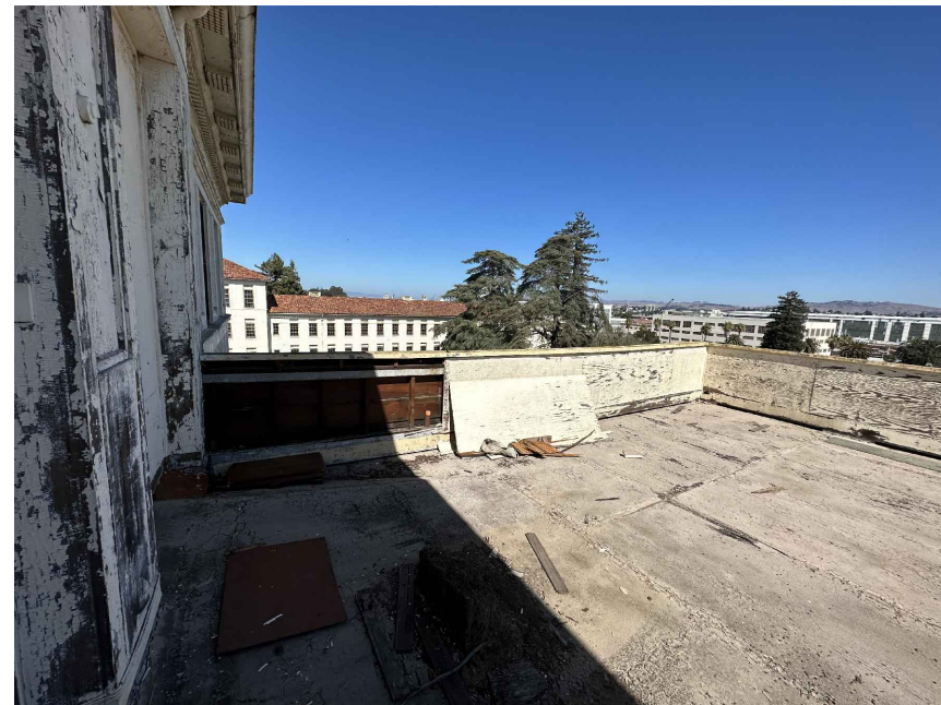
5 COLUMNS @ ROOF ENTRY
