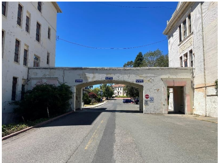
Figure 8. The arch bridge walkway connecting Building H1 and Building H80, view southwest.
