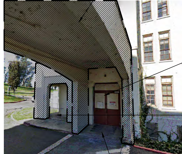
2 H1 NORTH WEST WING NORTH WEST VIEW
