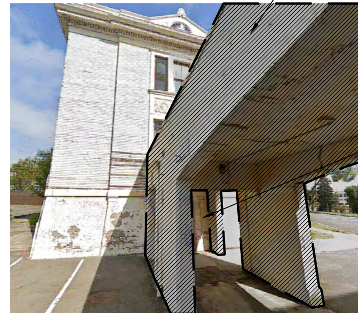
6 H1 MAIN BLDG SOUTH END SOUTH WEST VIEW
