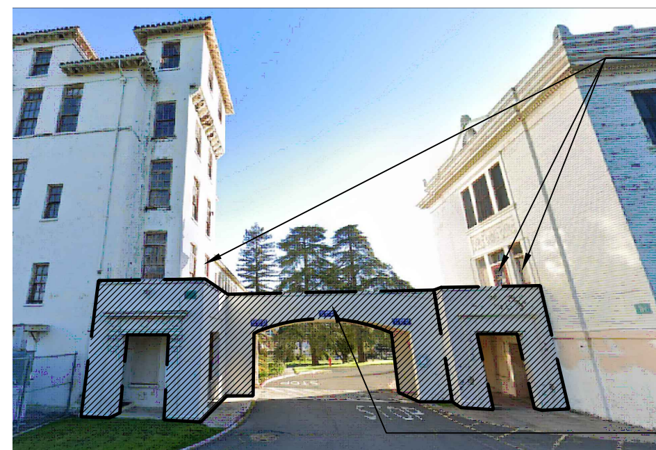
4 SOUTH WEST WING BRIDGE SOUTH WEST VIEW
