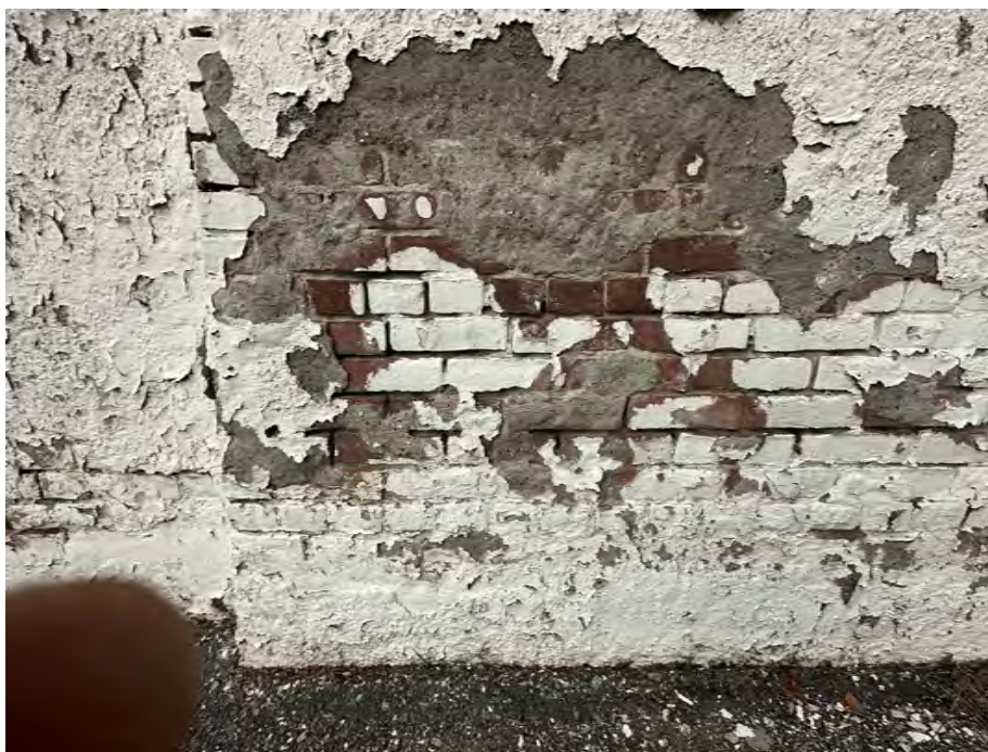
PLASTER REPAIR AND BRICK RESTORATION
